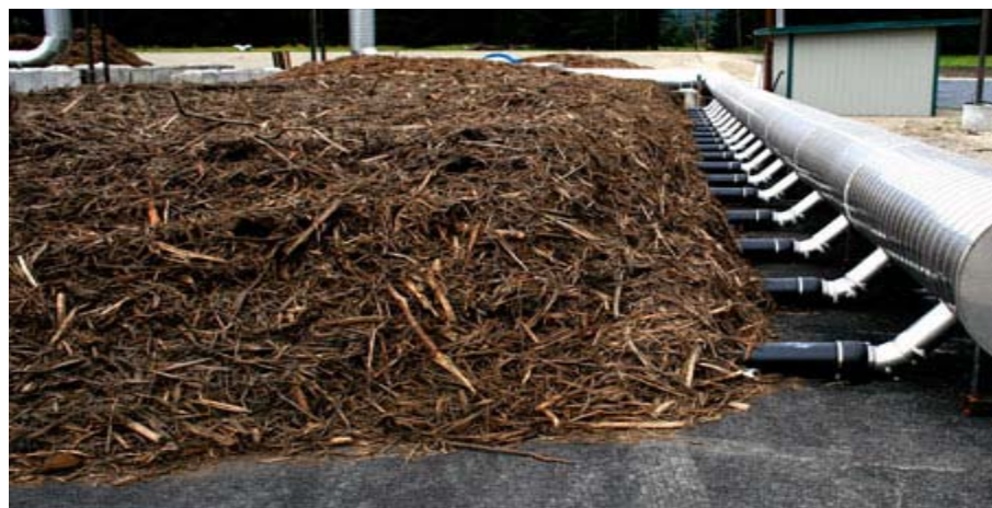
Typical ECS Biofilter designed for the AC Composter™>
