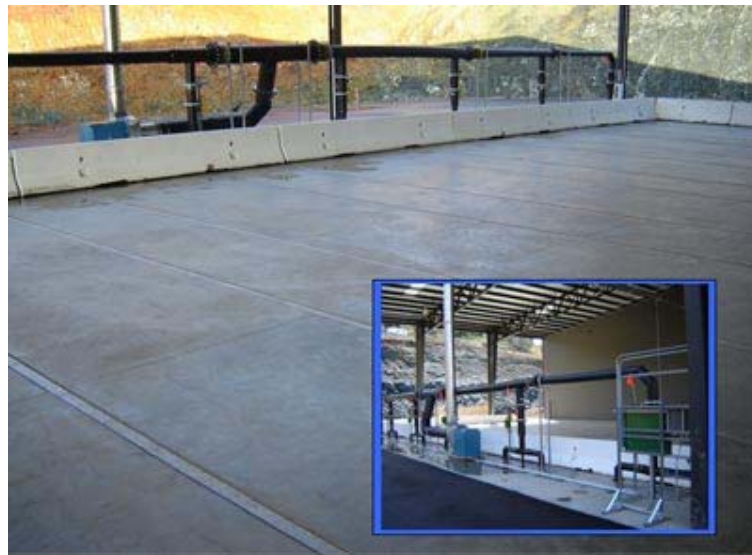
Mariposa County, CA Extended Curing ASP
