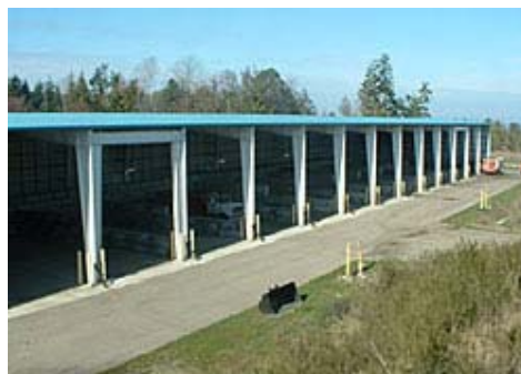
Biosolids Composting Facility Port Angeles, WA
