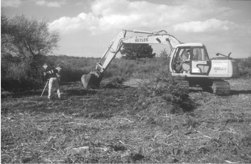
Fig 4. A caterpillar crane with flat shovel scrapes away woody debris, litter and part of the topsoil in a wet dune slack of De Westhoek (2000).
