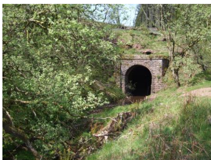
Former railway line, Talybont valley
