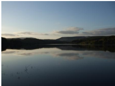
Llywn-onn Reservoir, completed in 1926
