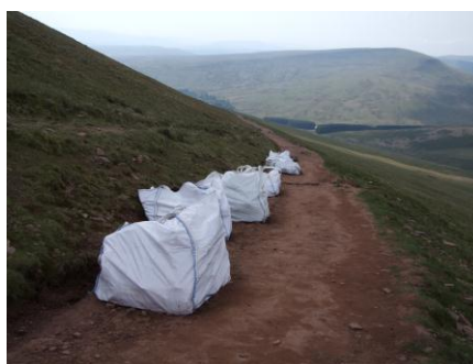
Bags of stone (dropped by helicopter) for pitching the popular path to Corn Du from Storey Arms.
