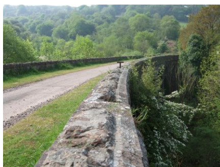
Woodlands and viaduct on valley side
