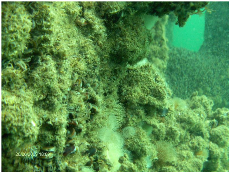
Picture 3: Marine growth on the monopile
