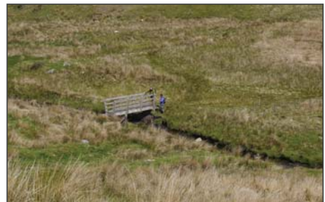
Footbridge over the Afon Disgynfa
