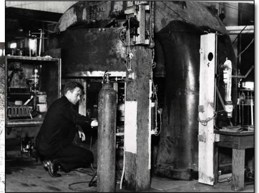
Lawrence at Work on the 37" Cyclotron, 1937, 8.5 MeV deuterons
