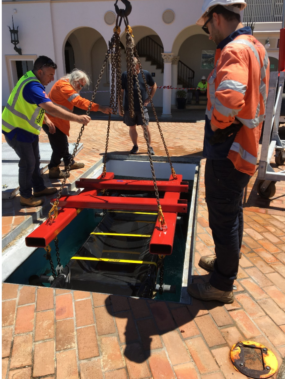
Figure 6. Lifting the stretcher through the hole cut above the med pool.
