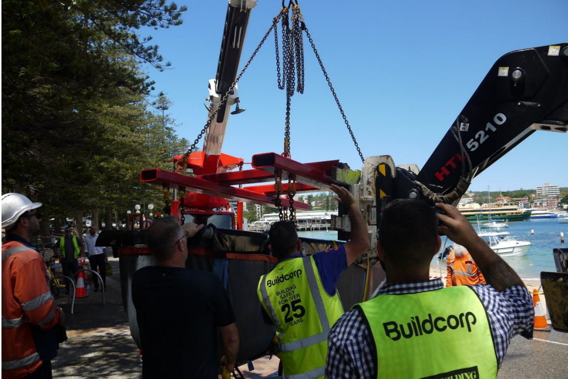
Figure 7. Transferring from the Franna Crane (right) to Telescopic Handler Forklift (left).
