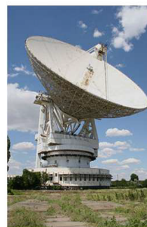
Fig. 2. The receiving and transmitting full-rotating antenna with a diameter of 70 m of the Center for Remote Space Communications in the Crimea, used for the USSR's planetary radar since 1980.
