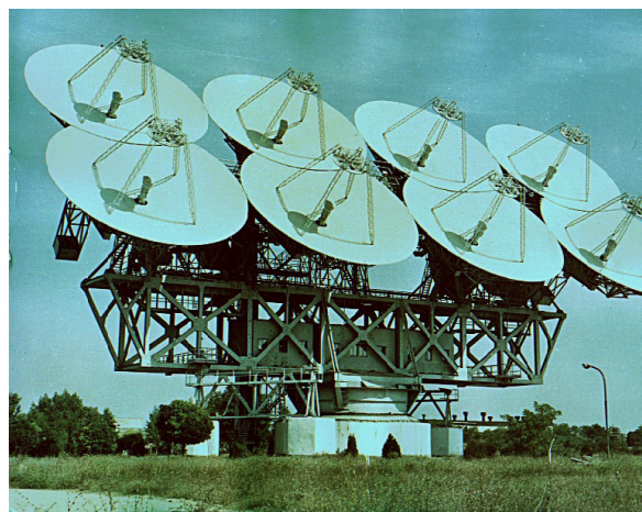
Fig. 16. Antenna of the Center for Remote Space Communications, used in the USSR's planetary radar prior to 1980.
