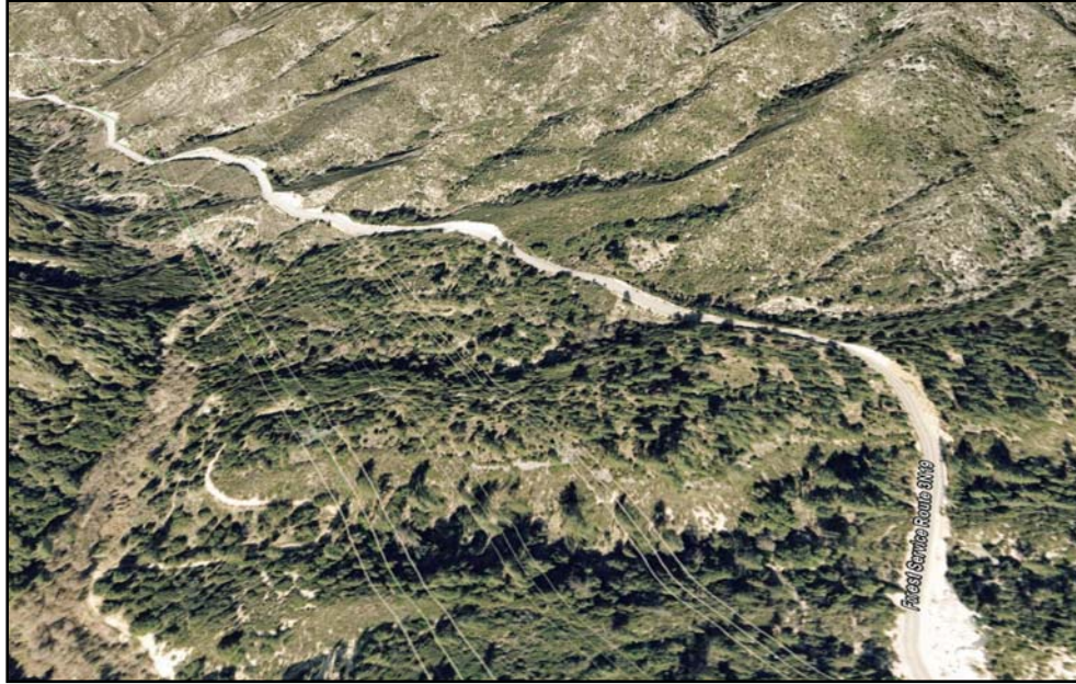
Photo 10: Aerial (oriented north) of potential shaft location where construction would switch from tunnel boring to cut/cover trench tunneling within Upper Big Tujunga Canyon Road (near S6 MP 16.0). Source: Google Earth.
