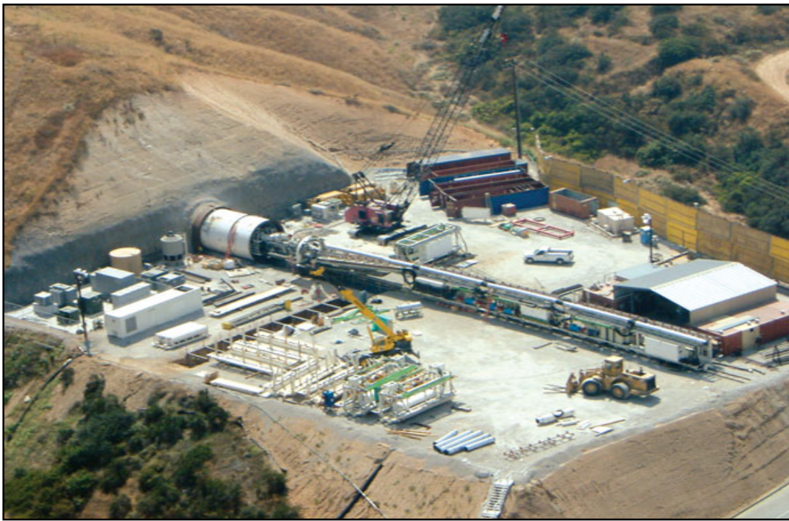
Photo 1: Assembly of the tunnel boring machine at the Strawberry Creek Portal. Source: Neufeld, 2007
