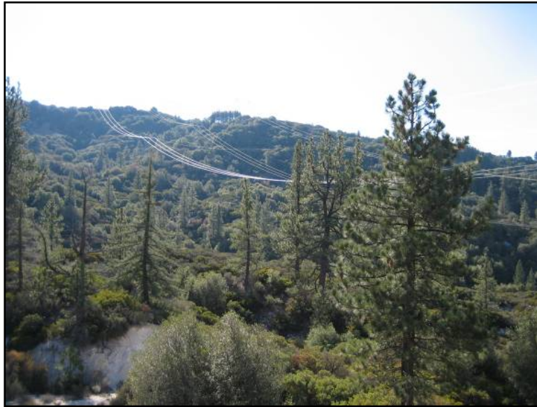
Photo 9: Looking south from Upper Big Tujunga Canyon Road towards Angeles Crest Highway (S6 MP 16.3).
