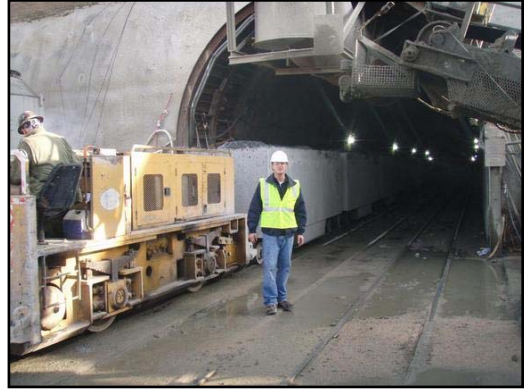
Photo 6: Rail car engine at Strawberry Portal. Source: LetsGetNuts.com, 2008.
