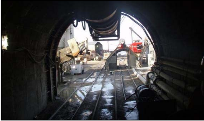
Photo 5: Strawberry Tunnel exit (City Creek Portal). Source: LetsGetNuts.com, 2008.
