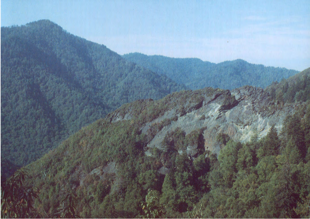
Figure 1.—An exposure of the Anakeesta Slate Formation as viewed from the Alum Cave Bluff Trail in Great Smoky Mountains National Park.
