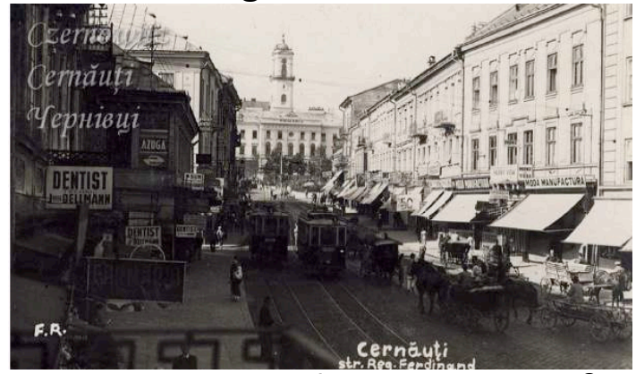
Former Enzenberg Hauptstraße
