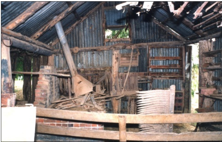
Blacksmith Shop interior & Forge 'as found'
