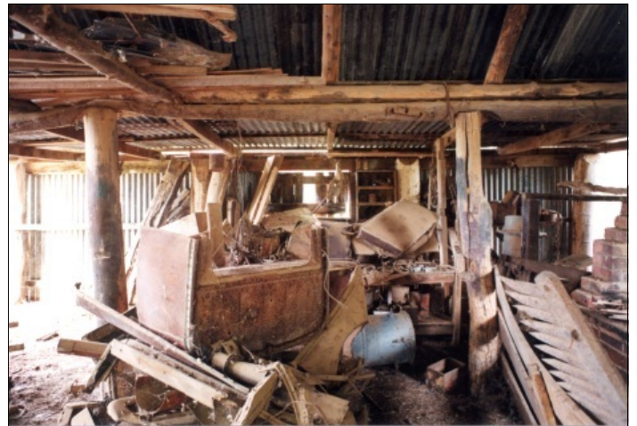
Blacksmith Shop interior 'as found'
