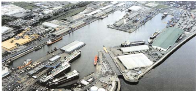
Hull—King George Dock and Queen Elizabeth Dock
