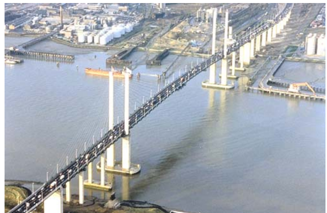
The Queen Elizabeth II Bridge
