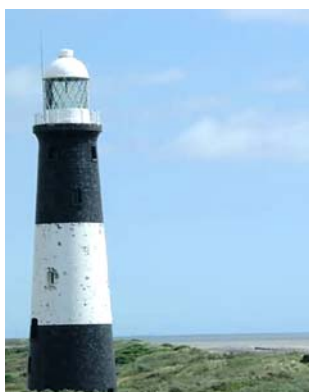
Spurn Head Lighthouse (disused)
