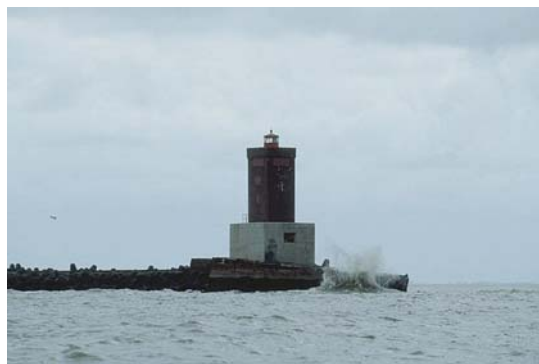
Minsener Oog Disused Light Tower (Buhne A)
