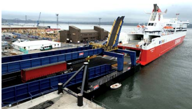
Rosyth Ferry Terminal
