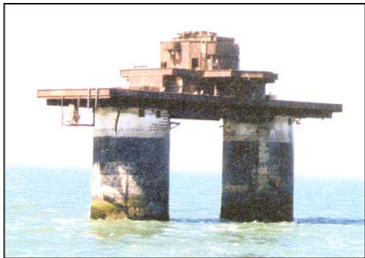
Knock John Tower
