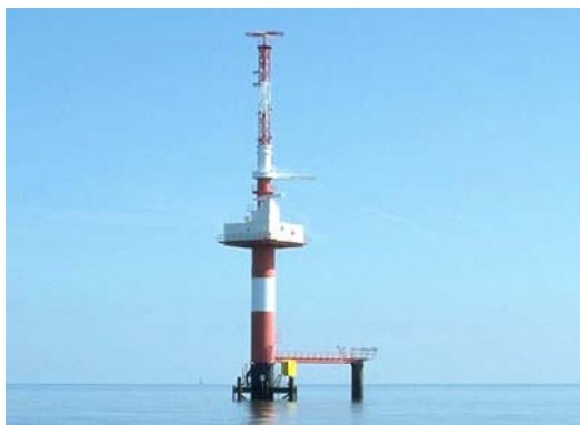
Hooksielplate Radar Tower
