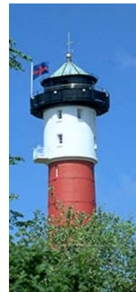
Wangerooge Disused Light Tower
