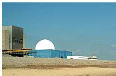
Sizewell Nuclear Power Station
