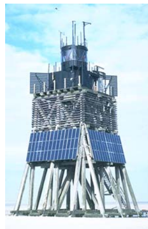
Suderoogsand Light (Refuge Beacon)
