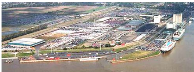
Emden Ro-Ro Terminal
