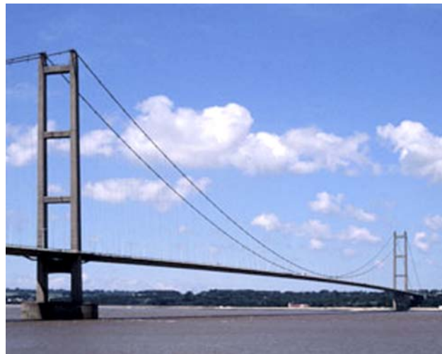
The Humber Bridge
