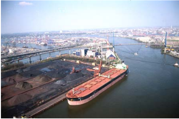
Hamburg Bulk Terminal
