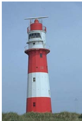
Borkum Little Disused Light Tower
