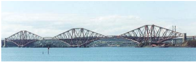
The Forth Bridges from NE
