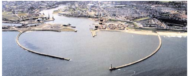
Entrance to the River Wear (Sunderland)
