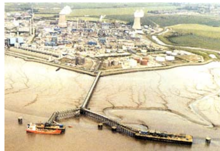
Salt End Oil Terminal
