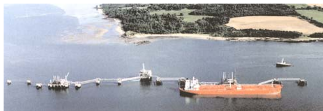
Hound Point Terminal
