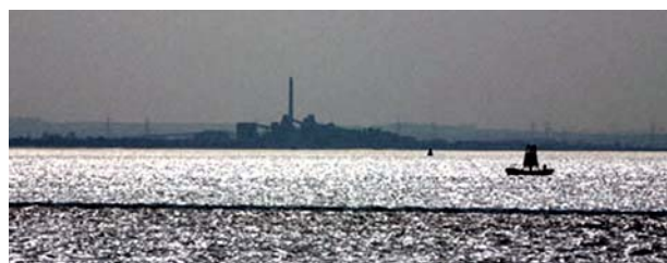
Ferriby Sluice (cement factory chimney)
