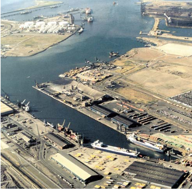
Tees Dock and Norseia Oil Terminal
