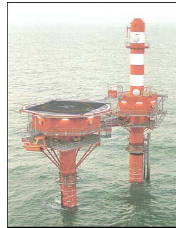
Oostdyck Radar Tower
