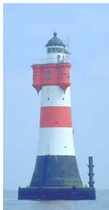
Roter Sand Tower
