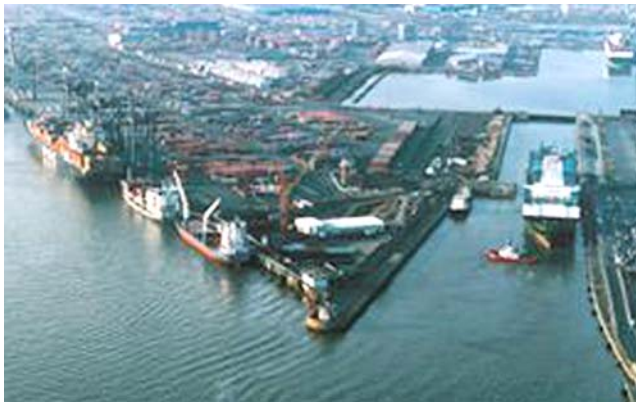
Bremerhaven—Nordschleuse (North Lock)
