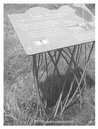
Grass-style base for the unframed sign panel. Sign panels are bolted into the back from a base plate which is welded to the grass-like aluminum rods.
