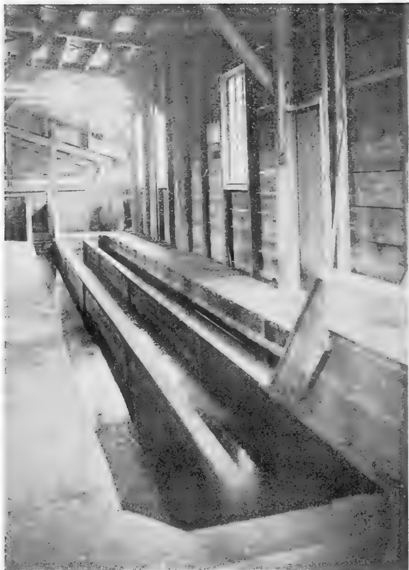
Mammoth Sheep-Dipping Vat at the New York Central Stock Yards, Buffalo, N. Y. Length of Swim in the clear 136 feet. Capacity 100 Sheep at a time. Heated by steam and with all the latest improvements, making it by far the largest and best appointed Dipping Plant in the United States.
