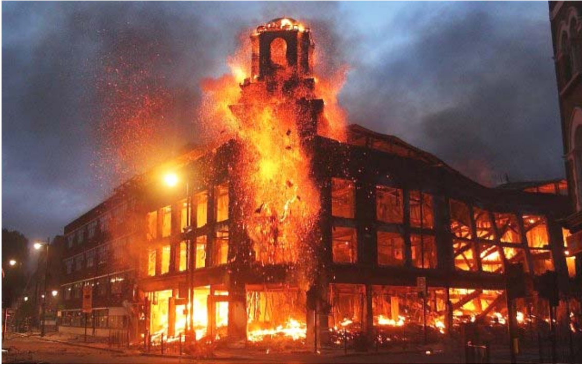
Fig. 1. Example the effect of fire to building structures
