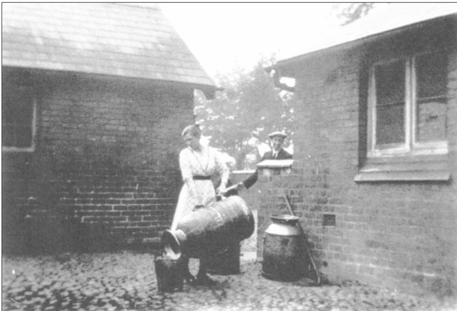
III. 20: Outbuildings at Leftwich Old Hall.
