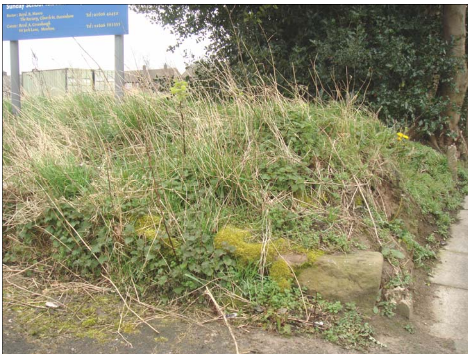
III. 36: Stone kerb on the south side of the entrance from Ellesmere Road.
