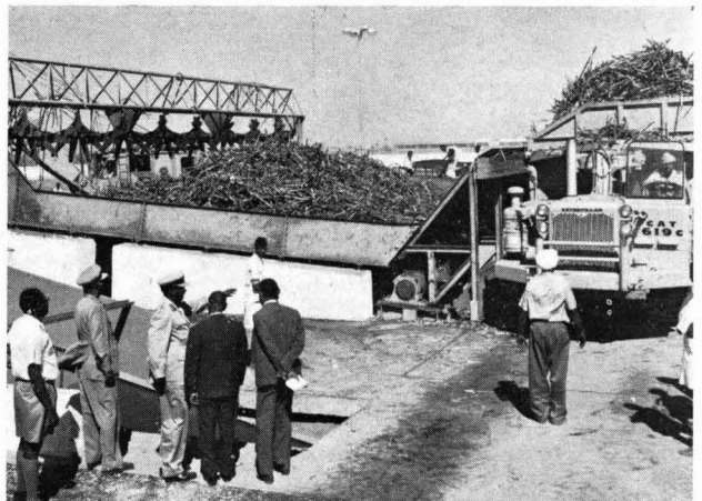
Fig. 2. Cane Feed Table with Hilo Cane Transporter; third man from left is Brigadier IBRAHIM ACHMED OMER, General Manager of the Guneid Sugar Factory.
