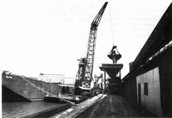
Fig. 1. Raw sugar unloading at Redpath Sugars Inc.
