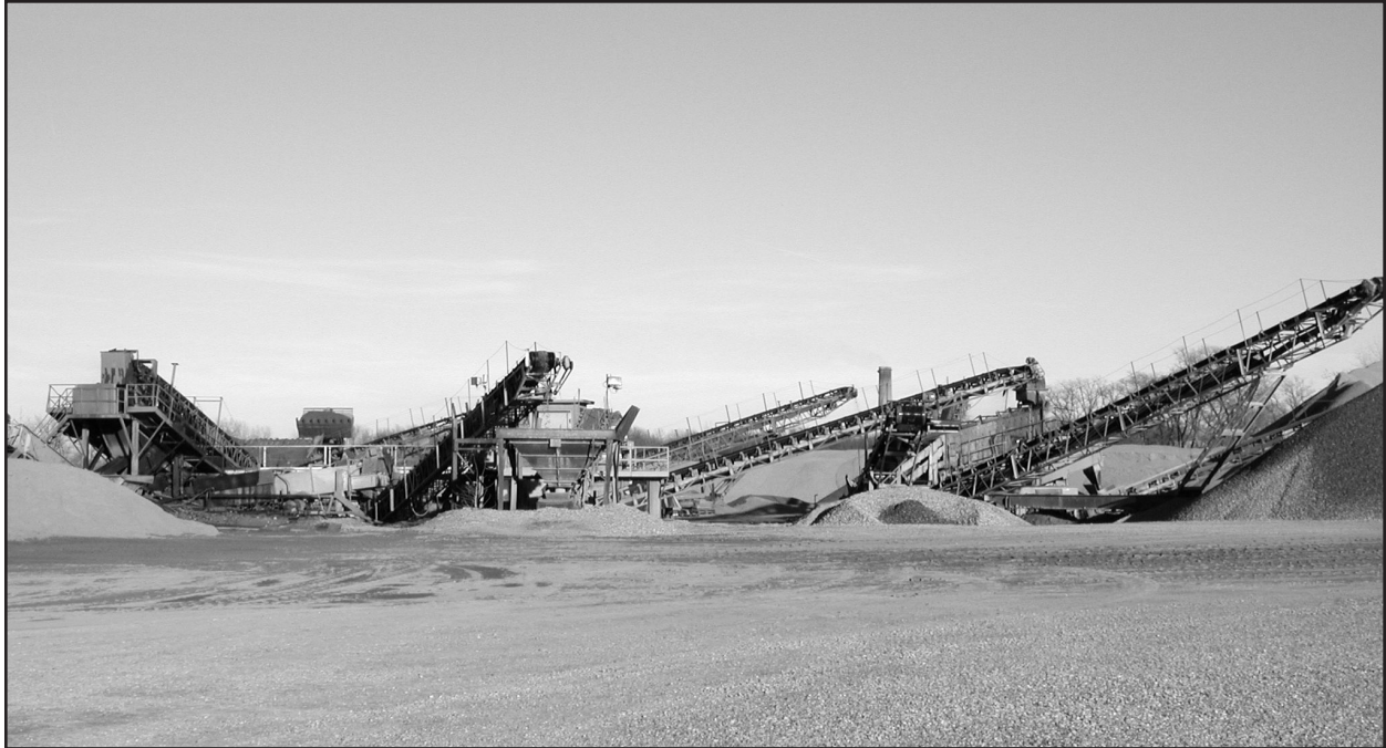
Figure 22 Preparation plant at Cornick Sand and Gravel Pit at Stop 6 (photo by W.T. Frankie).
