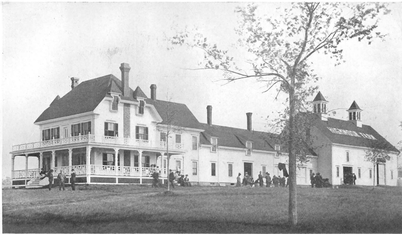
HIGHMOOR FARM BUILDINGS
