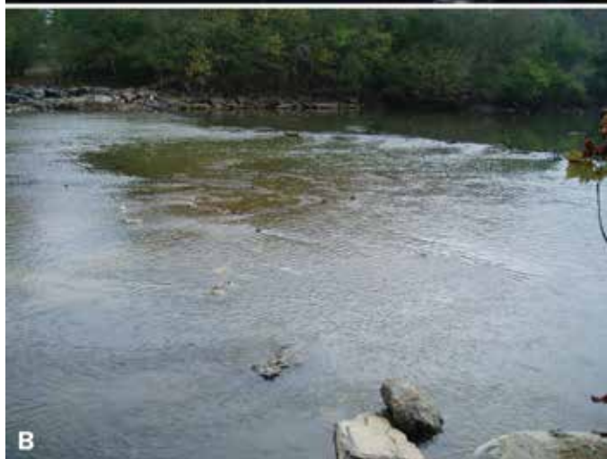
Figure 6. (A) Former Marvel Bridge located in the Cahaba River north of the Cahaba National Wildlife Refuge. The bridge (slab) was constructed by a mining company in the 1970s to move coal across the river and remained after the mine closed. (B) Efforts by the Nature Conservancy of Alabama culminated in its removal in late 2004, which improved habitat conditions over a kilometer of river and eliminated a barrier to fish passage. Photo Credit: Paul Freeman, the Nature Conservancy of Alabama.
