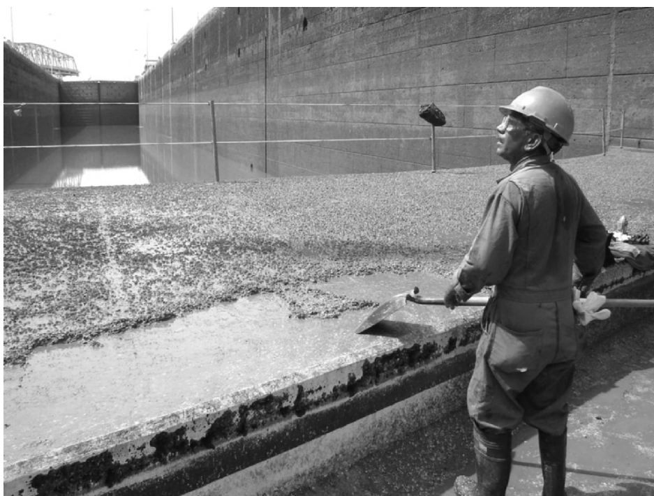
Fig. 6. Barnacles being scraped from the bottom of Miraflores Lock during draining in 2005. Photo courtesy of Mark Torchin.
