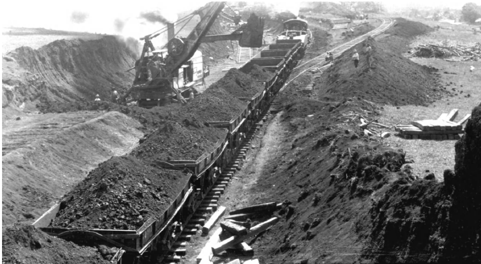
Fig. 9. Moving the dirt. Photo courtesy of the Panama Canal Authority.
