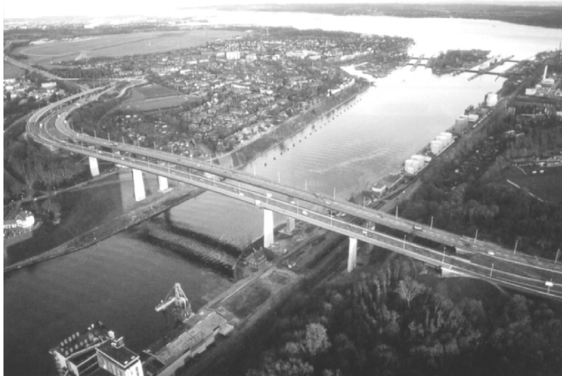
Fig. 22. Aerial view of the canal bridge and locks (background) in Kiel-Holtenau. Photo courtesy Klaas Hinderk Rosenboom, Hamburg, Germany.
