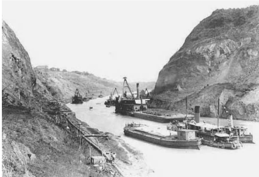
Fig. 10. Floating dredges at work in the Culebra Cut. Photo courtesy of CanalMuseum.com.
