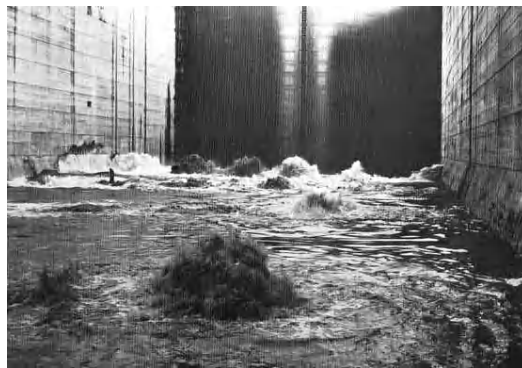
Fig. 4. The first flooding of Miraflores Locks, with water entering through wells in the floor of the chamber. Photo courtesy of CanalMuseum.com.
