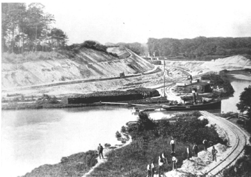
Fig. 9. Kiel Canal construction site (in the background) in 1892 with the Eider Canal in the front. The train tracks crossing the Eider Canal were needed to allow the construction works of the Kiel Canal. Photo courtesy of Walter Schulz, Brunsbüttel, Germany (Schulz 1995).
