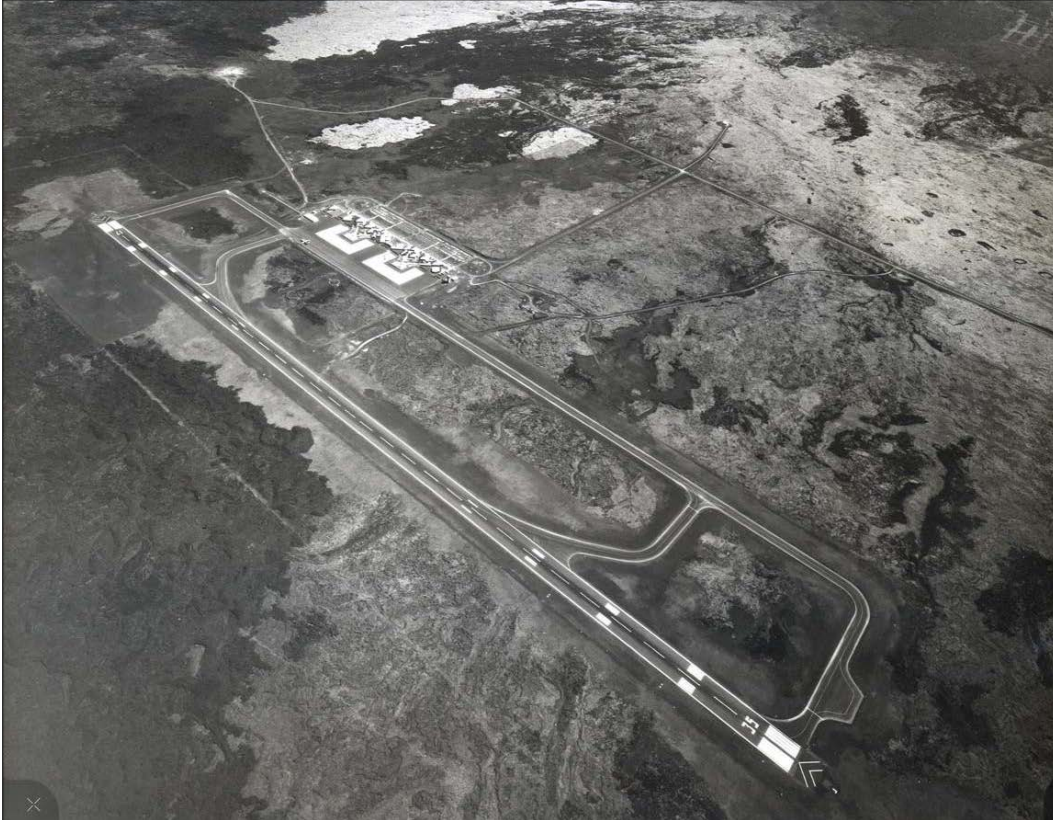
Figure 37. Oblique aerial view of the completed Keāhole Airport facility taken on October 6, 1971.
