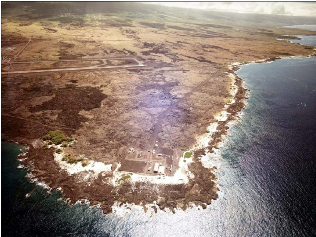
Figure 40. Oblique aerial view of the initial NELH facilities under construction in 1980.
