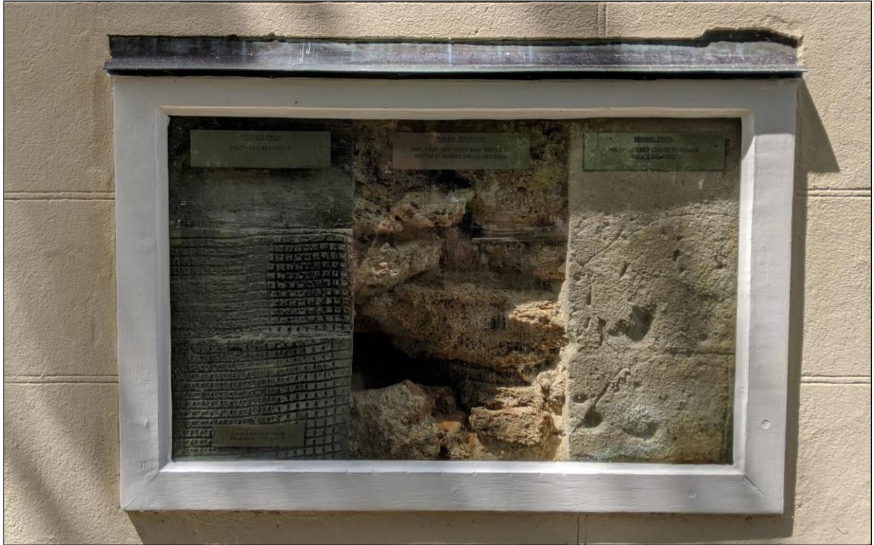
Figure 24. The preserved wall at Grace Episcopal Church. Original shell hash is visible in the center section (NPS/MACKENZIE CHRISCOE).
