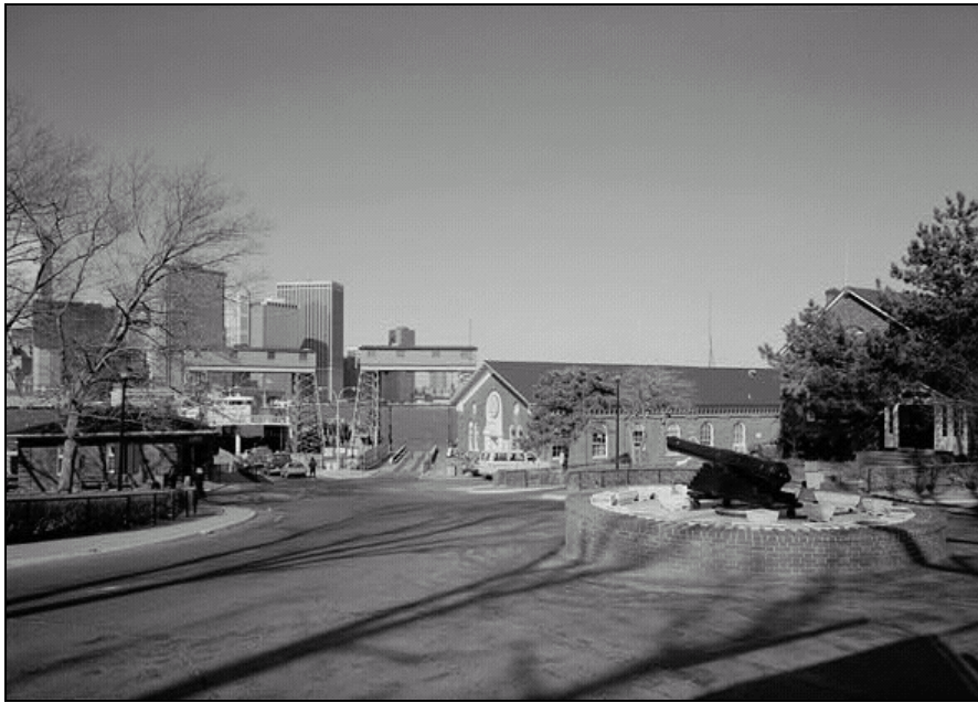
Figure 35. Building 140 is in the center of the photograph, next to the ferry slip. HABS-HAER Report.
