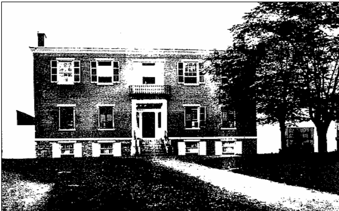
Figure 21. Building 9 Post Hospital, 1864 Photograph. HABS-HAER Report.
