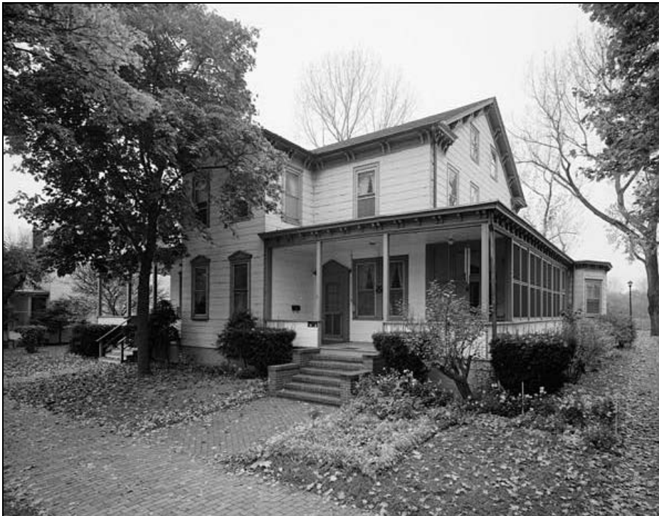
Figure 32. Building 19, a duplex built to standard plans. HABS-HAER Report.
