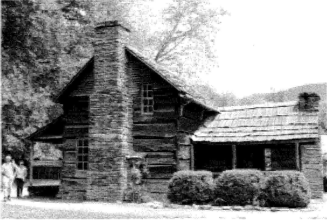
Figure 3: Joe Queen House, looking east- 2012
