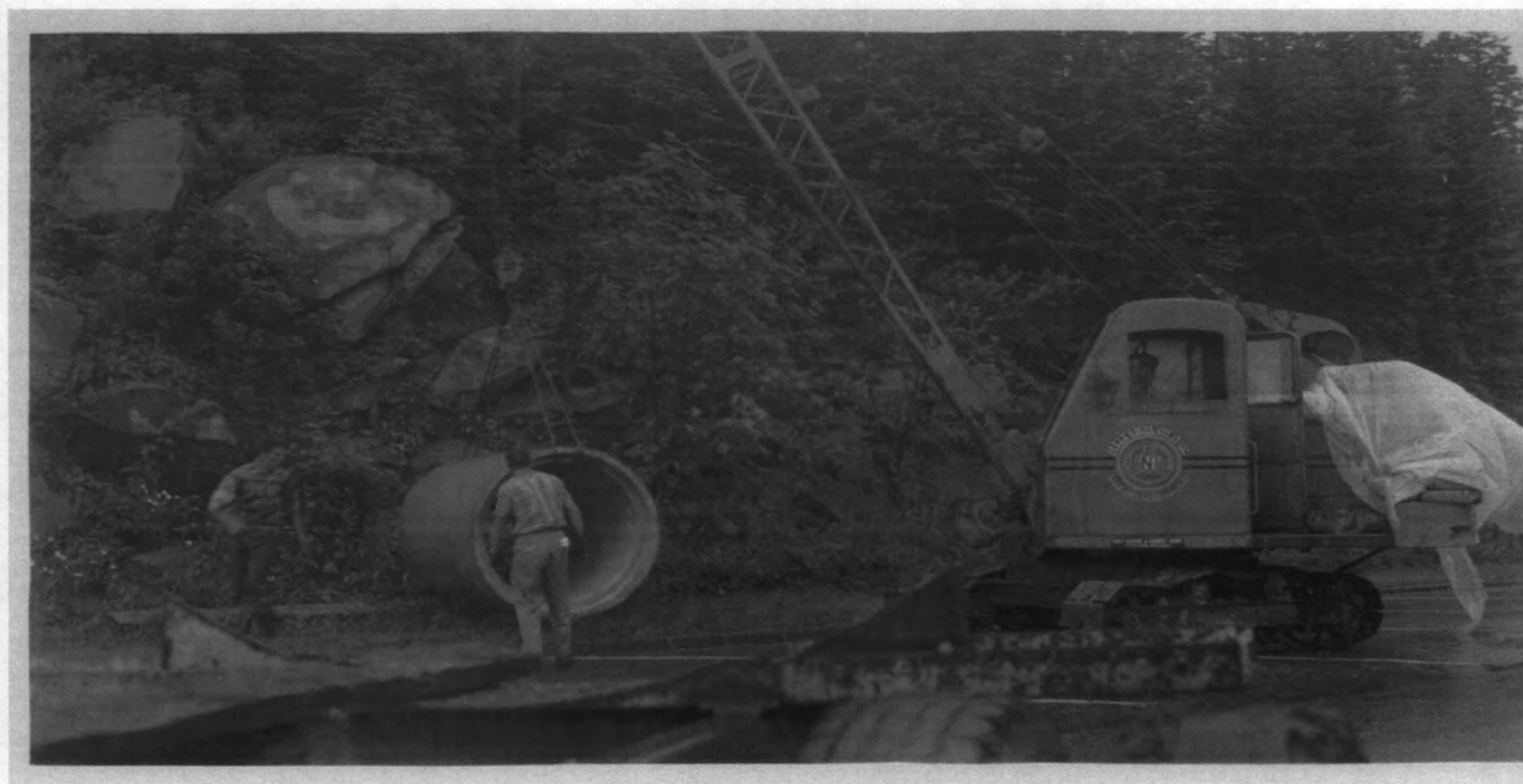
Fig. 7 "Loading Sections of Main Column at Clingmans Dome" NPS photograph by R.A. Wilhelm, 1959. Archives of GRSM.
