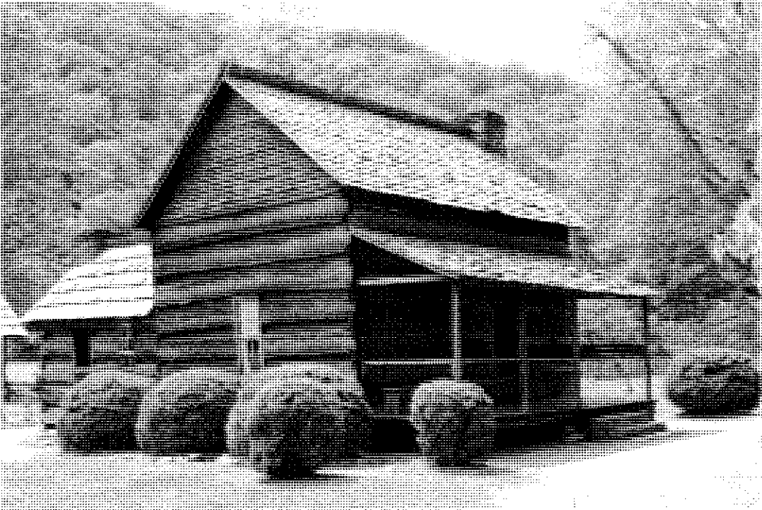
Figure 1: Joe Queen House, looking west- 2012
