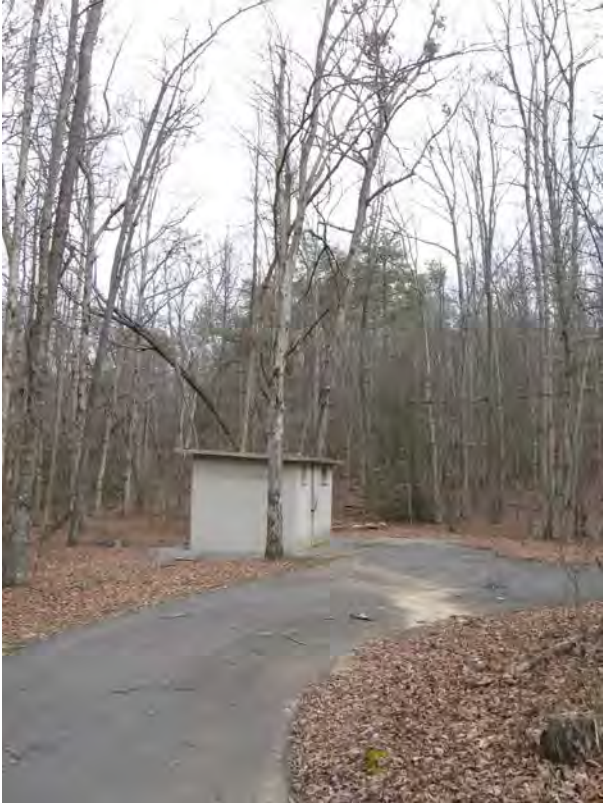
Water Pump House Station (2012)
