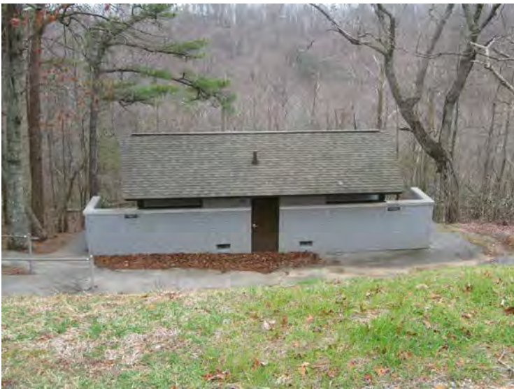
Picnic Area Comfort Station (2012)
