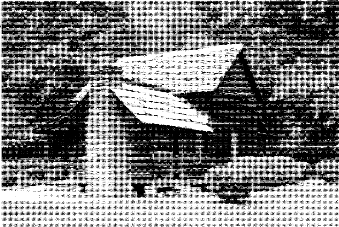
Figure 2: Joe Queen House, looking northeast- 2012
