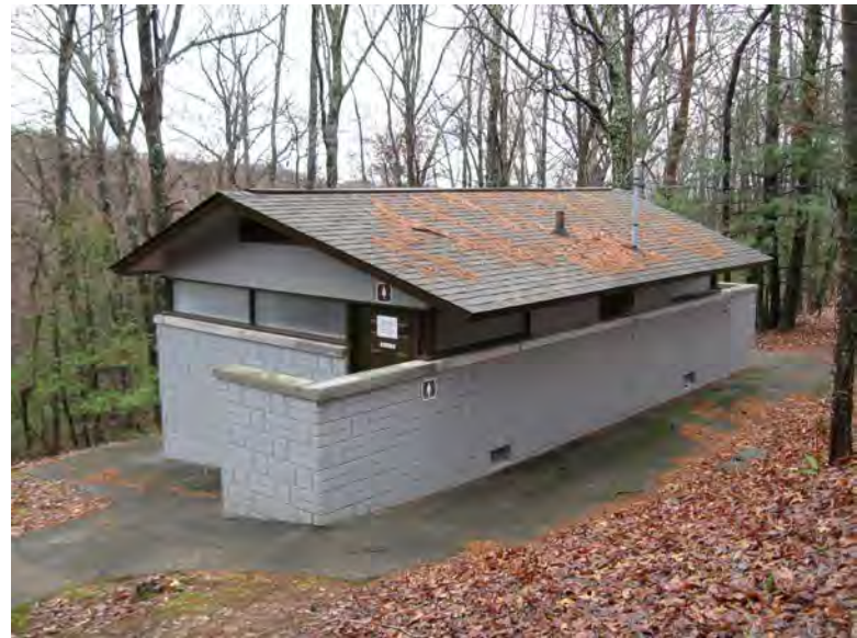
Campground Comfort Station (2012)
