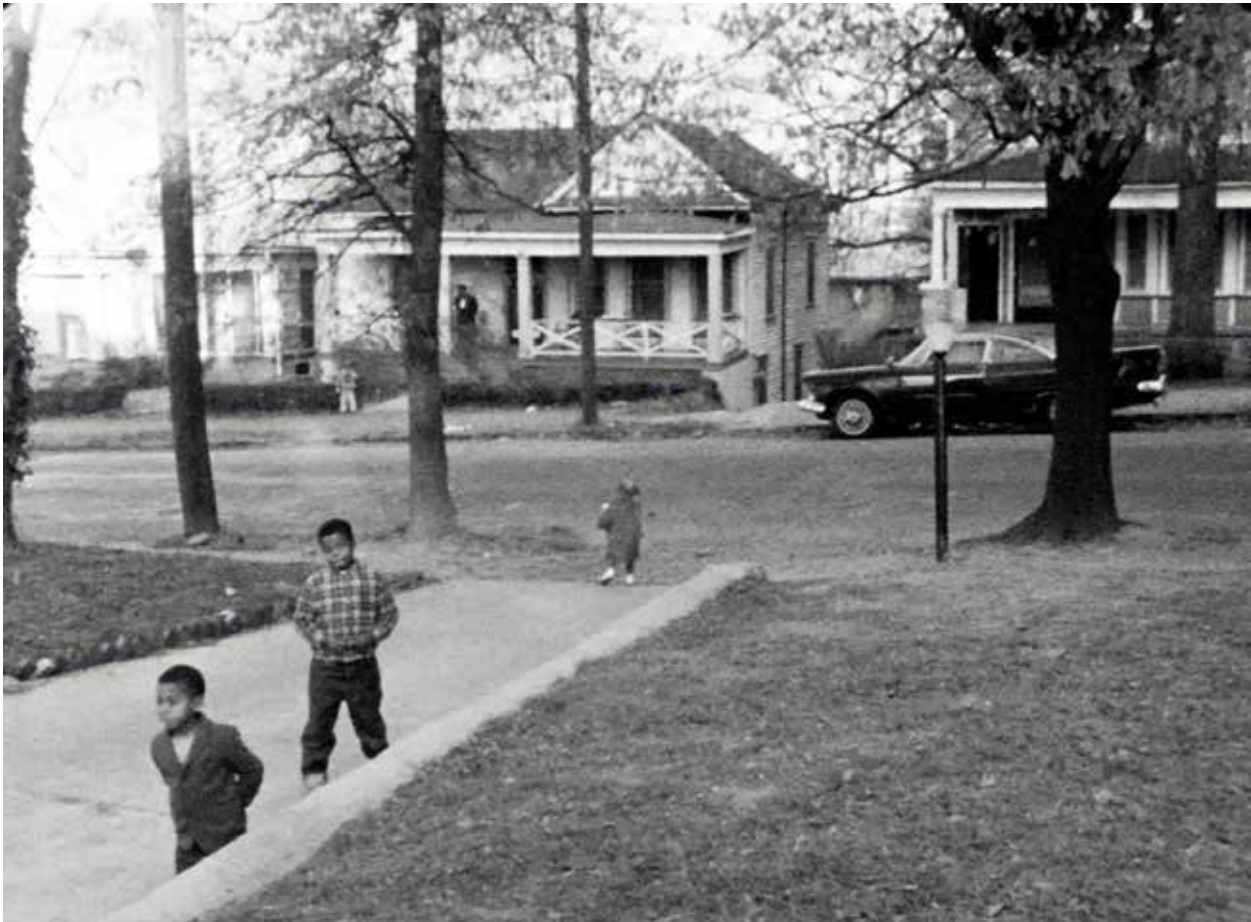
Figure 2.56. December 1965 view of the front yard and driveway, facing northeast. (Source: MLK and Arnold Michaelis Interview, Raw Footage Reel 8, University of Georgia, Peabody Archives.)
