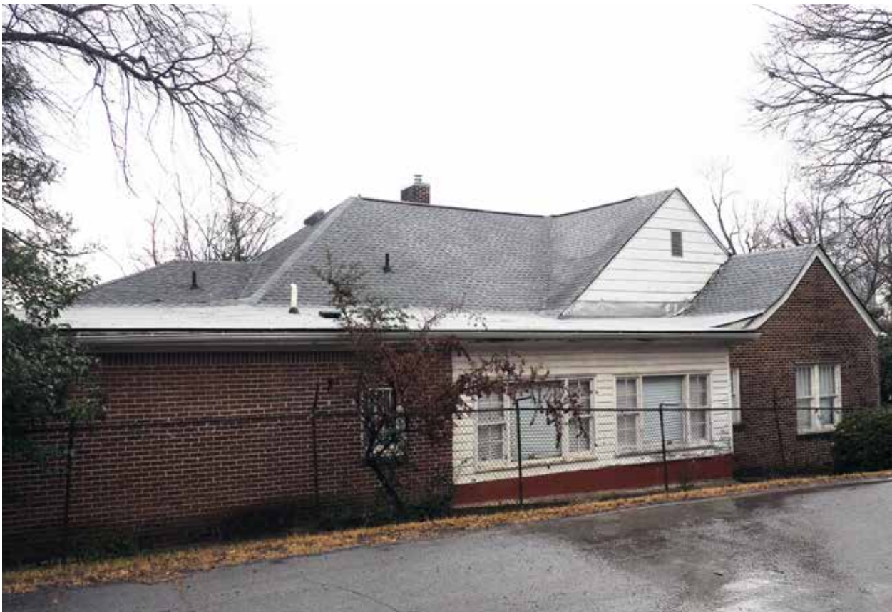
Figure 3.44. View facing northeast of the south elevation showing cross-gable roof of main house rising above the south elevation one-story low slope extension. (Source: WLA Studio, January 2021.)
