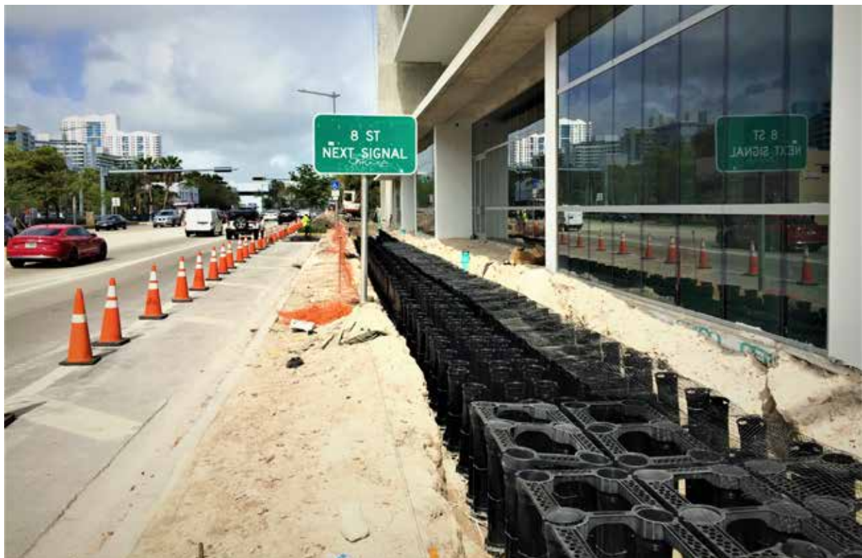
Figure 5.2. View of installation of a modular suspended pavement system. (Source: © 2021 Deeprout, deeprout.com.)
