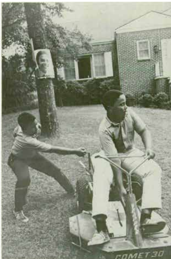
Figure 2.65. Martin Luther King III (on mower) and Dexter (starting mower) in front yard, 1970. Note the evergreen foundation plantings are still present in front of the house, and vegetation has increased near the southeast corner of the house. (Source: Ebony – permission pending, see Appendix E.)
