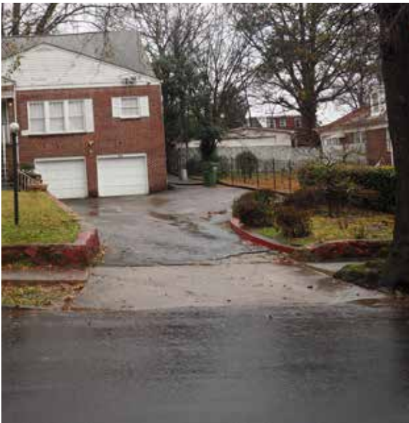
Figure 3.12. View of the asphalt driveway on the northeast section of the property, facing west. The driveway is lined by the stone retaining wall on the south and a concrete curb on the north. The apron leading from Sunset Avenue is concrete. (Source: WLA Studio, June 2020.)
