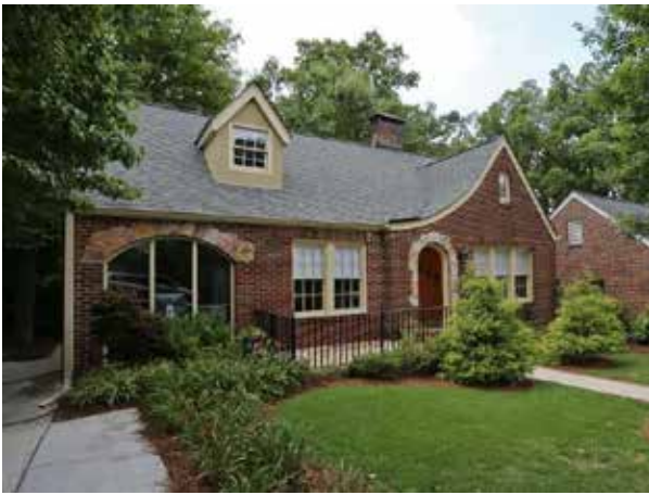
Figure 2.23. Chester R. Elliott House (1935), 911 Highland Terrace NE, Atlanta. The right-hand three bays appear to be a close match to the King Family Home's original appearance. (Source: Realtor.com, 2019.)
