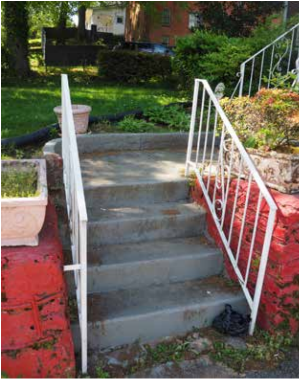
Figure 3.17. Three concrete risers with decorative metal handrails connect to a concrete walkway, facing south. (Source: WLA Studio, June 2020).
