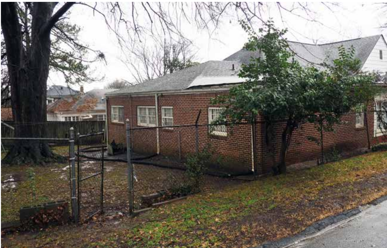
Figure 3.63. View of the chain link fence near the southwest property corner, facing northeast. (Source: WLA Studio, April 2020.)
