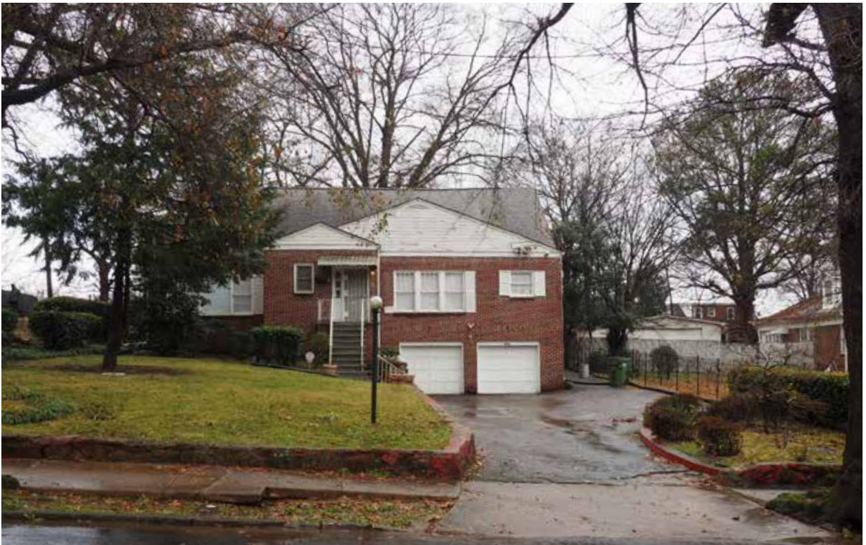
Figure 4.14. View of King Family Home from the east side of Sunset Avenue. (Source: WLA Studio, June 2020.)
