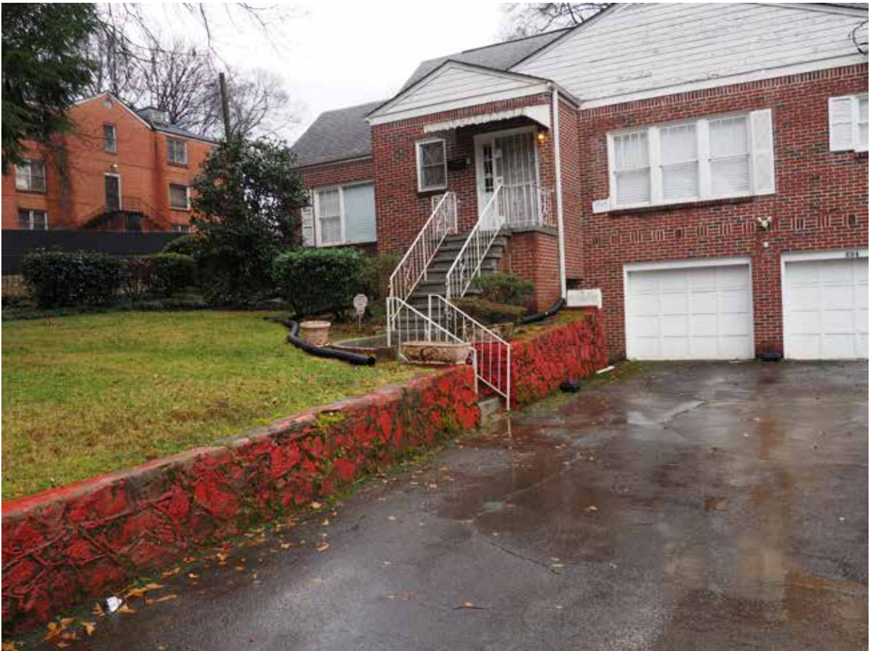
Figure 3.21. View facing southwest showing how the natural grade has been excavated to accommodate the asphalt driveway and residence. Concrete staircase and walkway connect the driveway to the main entry of the King Family Home. (Source: WLA Studio, June 2020.)
