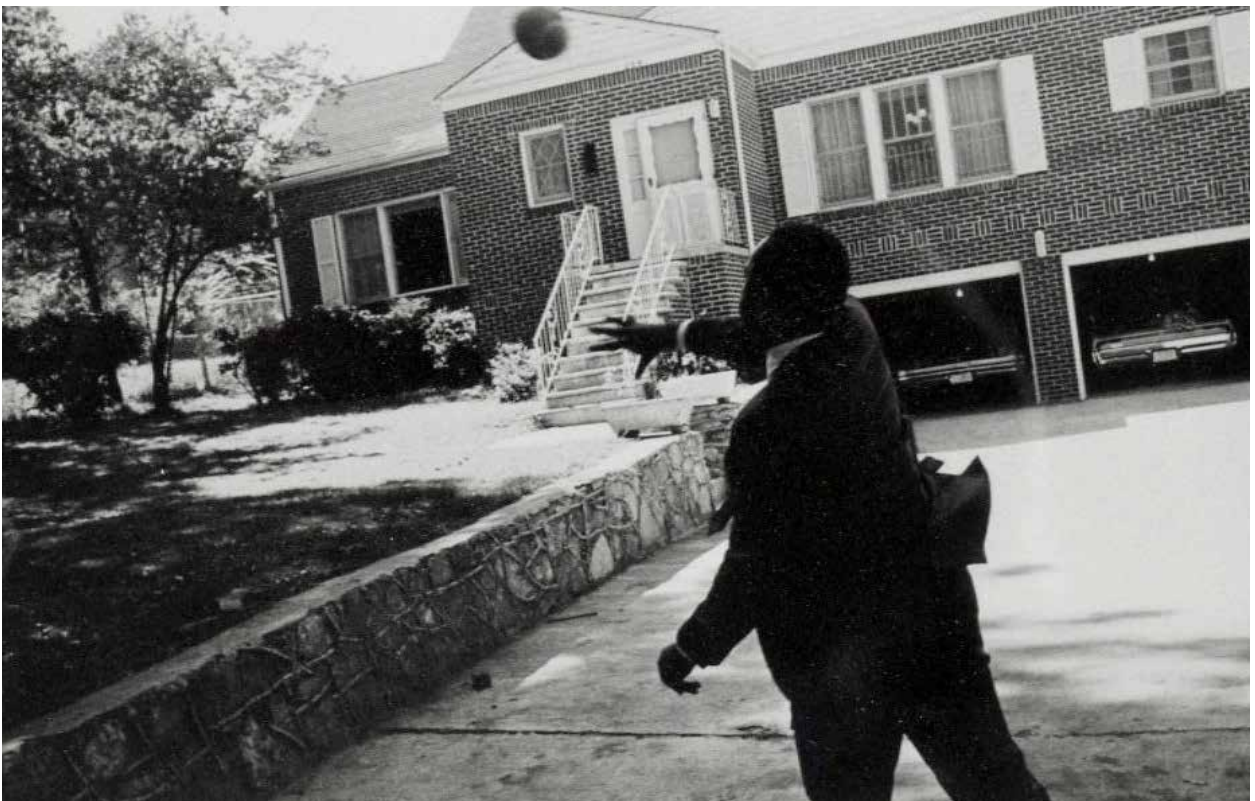
Figure 2.61. Undated photograph of Martin Luther King, Jr. in front of the King Family Home. View of the retaining wall and expansion joint in the driveway concrete. Evergreen shrubs are located at foundation. Unidentified trees are visible along the southern property line. (Source: MALU Archives.)
