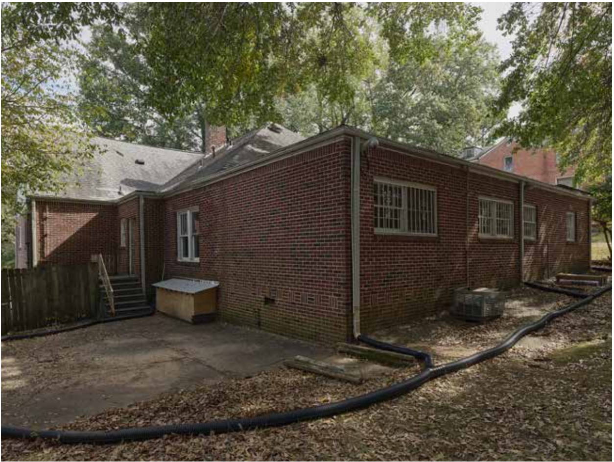
Figure 3.41. North and west elevations, facing southeast from rear yard. (Source HABS 199-8, October 2019.)
