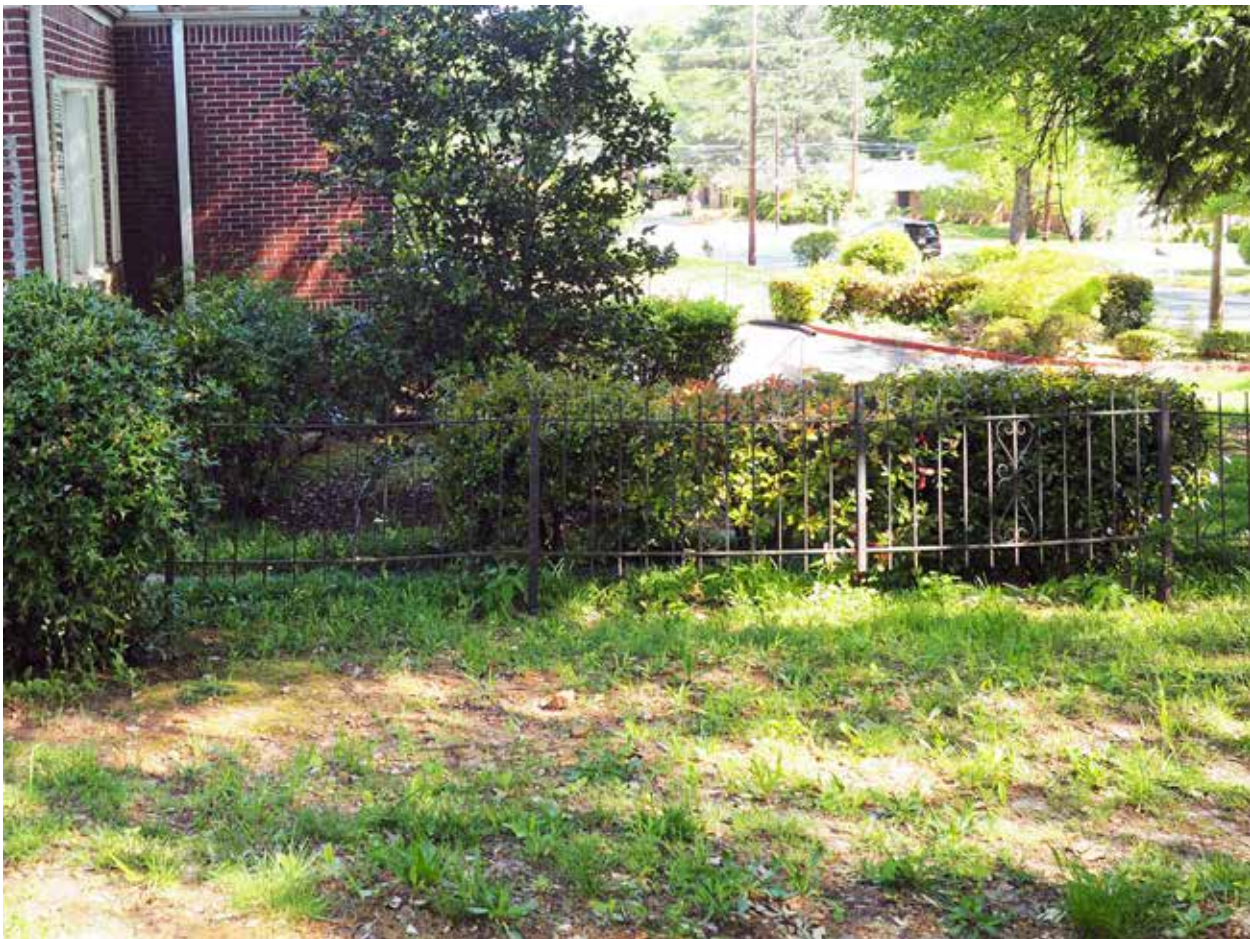
Figure 3.60. Anodized aluminum pike fence on the south side of the front yard, facing north. (Source: WLA Studio, 2020.)
