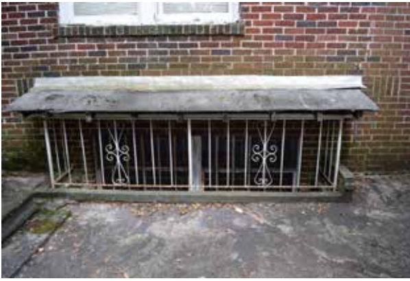
Figure 4.13. View of window well prior to plywood structure construction. Window was enclosed with plywood and flashing between June and October 2019 to reduce the amount of water ingress to the basement and the window well area. (Source: HPTC, October 2019 and WLA Studio, June 2019.)
