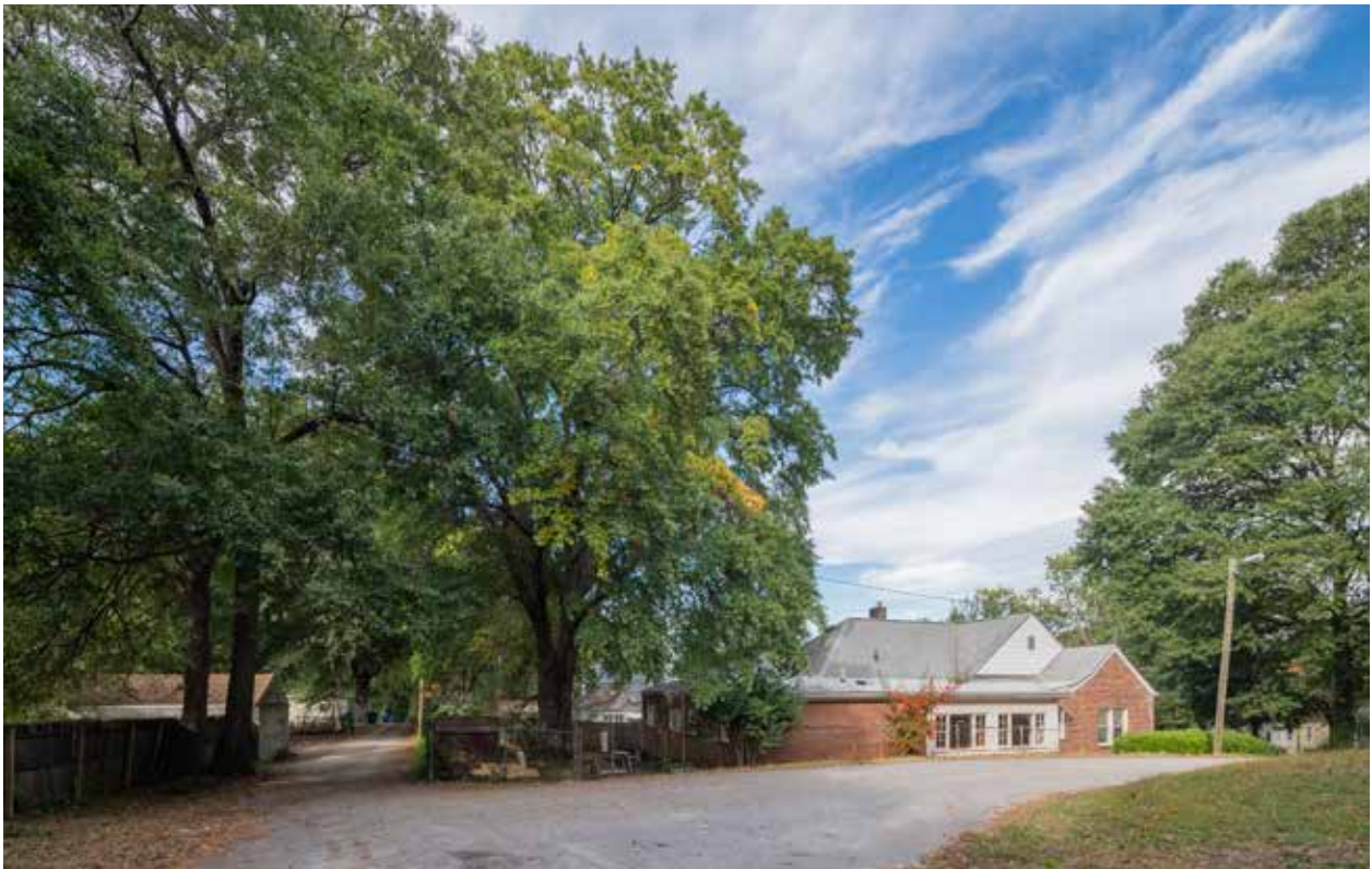
Figure 3.15. View of Dunkirk Street, located south of the property, and the alley, located west of the property, facing northeast. (Source: HABS_GA-199-7, 2020.)
