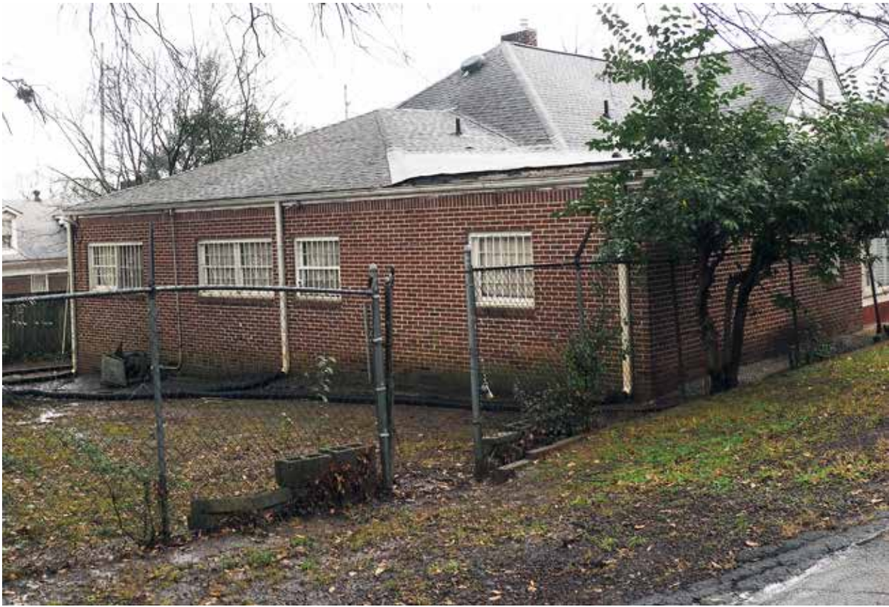
Figure 3.43. Oblique view facing northeast of the southwest corner of the residence. (Source: WLA Studio, January 2021.)
