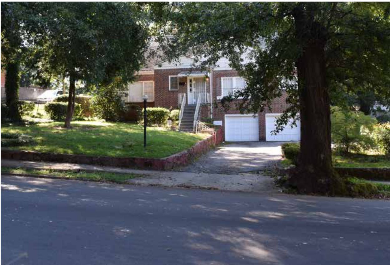
Figure 4.10. The house and retaining wall are intact at the site. The top photo is from 1965 and shows the retaining wall as constructed during the first house renovation. The lower photo is from 2020, and shows the later (1968) wall addition, which runs parallel to Sunset Avenue. (Source: MLK and Arnold Michaelis Interview, Raw Footage Reel 8, University of Georgia, Peabody Archives and WLA Studio, June 2020.)
