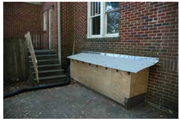
Figure 4.13. View of window well prior to plywood structure construction. Window was enclosed with plywood and flashing between June and October 2019 to reduce the amount of water ingress to the basement and the window well area. (Source: HPTC, October 2019 and WLA Studio, June 2019.)
