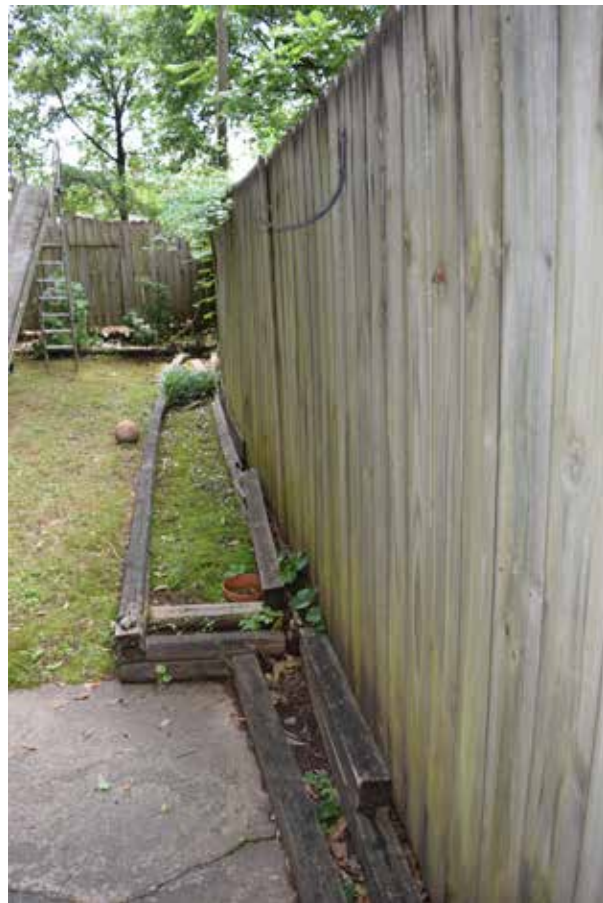
Figure 3.65. Raised landscape beds constructed from landscape timbers in the back yard. (Source: WLA Studio, June 2020.)
