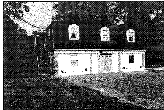
J. Garage/ Apartment, mid-twentieth century. View from the east.
