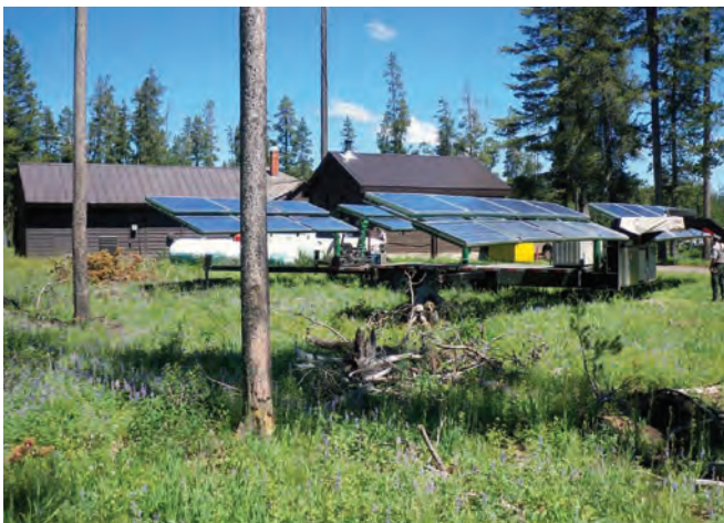
This portable photovoltaic system at Bechler provides power during the summer season, meeting 90% of the site’s electrical needs.
