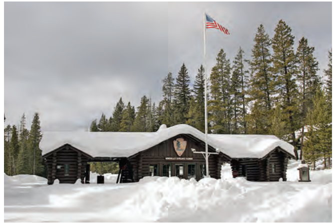
Northeast Entrance station is considered "the best of its type remaining in the National Park Service."
