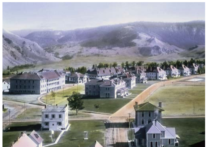
The irrigation system used to water the historic lawns of Fort Yellowstone and Mammoth Hot Springs, pictured here in 1916, was upgraded to include smart controllers which measure moisture levels.
