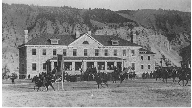
Albright Visitor Center, part of the Mammoth Hot Springs Historic District and Fort Yellowstone Historic Landmark District, housed the first "information office" (visitor center).
