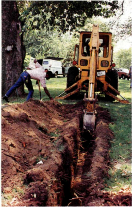
Figure 14. Trenching for disruption of root grafts between adjacent elms.
