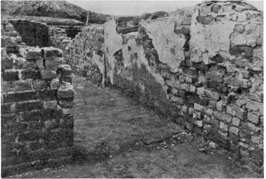
Interior wall of first statehouse foundations showing plaster fragments.
