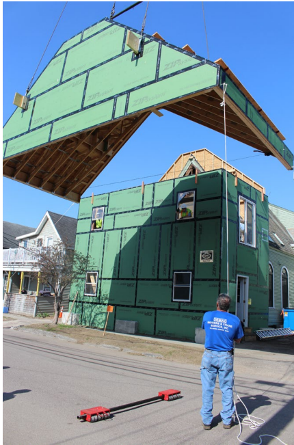
Left: Removing the roof at the Hyde St. location
