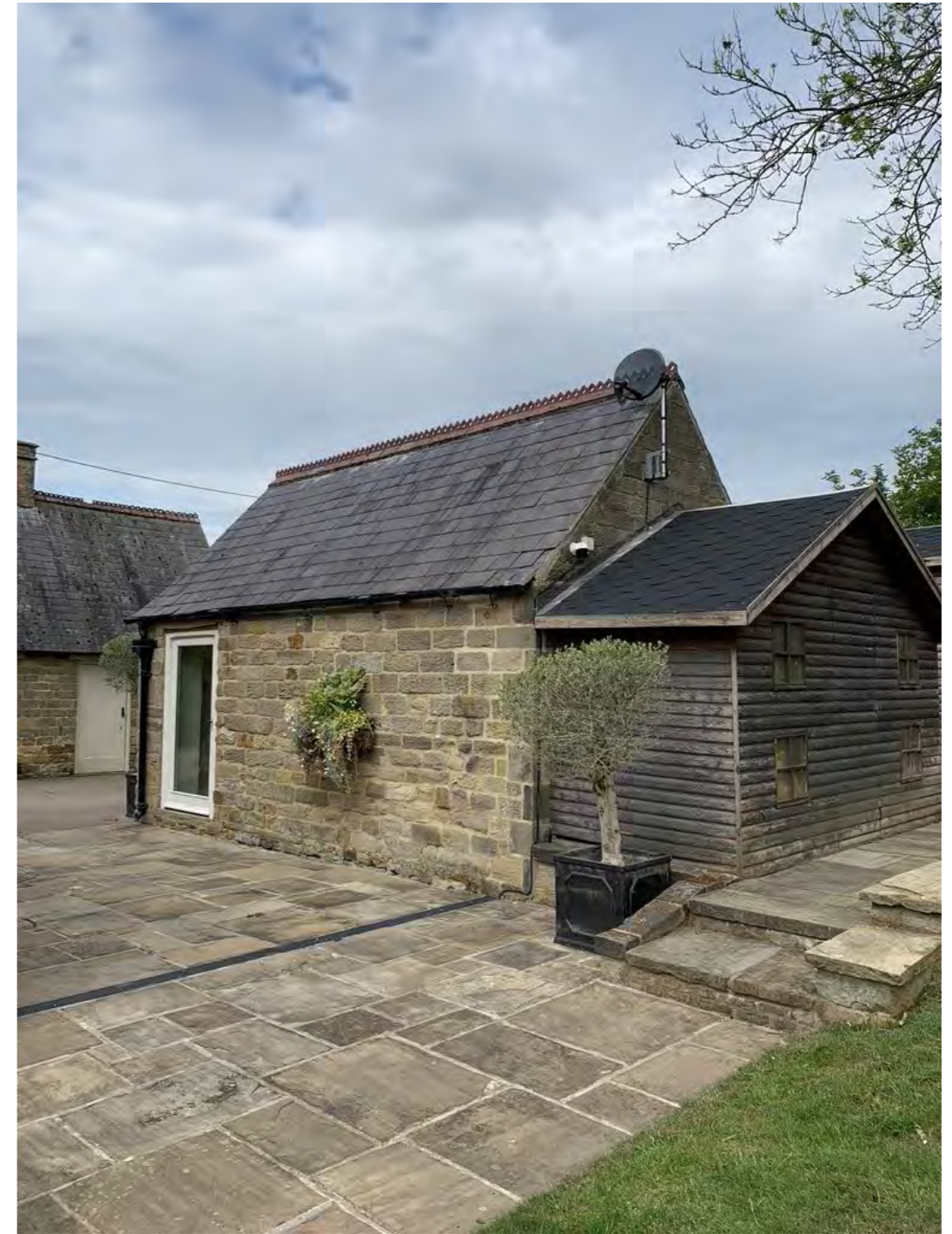
c) view of the south & north east elevations of the existing ancillary building currently being used as a gym. Proposal to retain the south wall and build new building and extend to the right hand side and back
