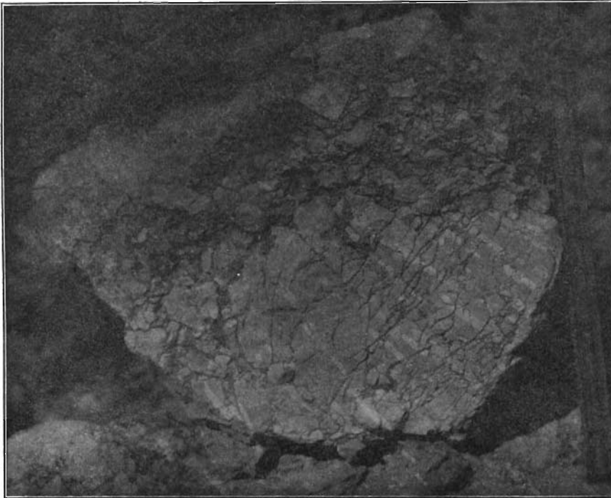
FIG. 61.—Block of massive Lower Davenport limestone, in part cracked, in part crushed to rubble. Felton creek, Cedar Rapids, Linn county.
