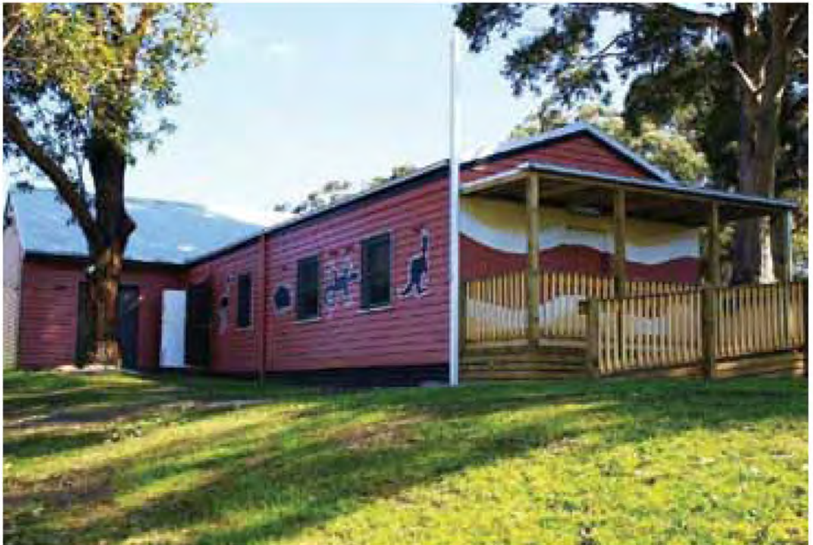
Kommel Koori Gathering Place: an old scout hall renovated for use as a community centre by participants in the Koori Offender Support and Mentoring Program in Morwell.
