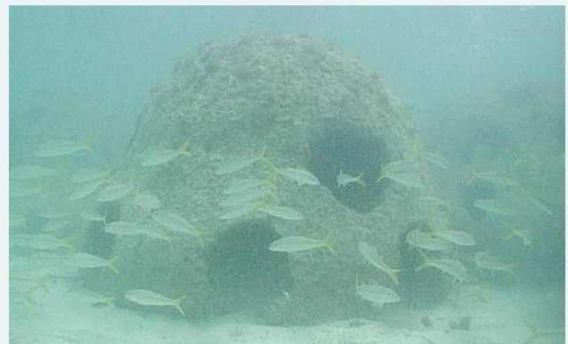
FIGURE 8 | Reef ball submerged breakwater for shoreline stabilization in Dominican Republic (1.2-1.3 m high, in water depths of 1.6-2.0 m) (Harris 2009).
