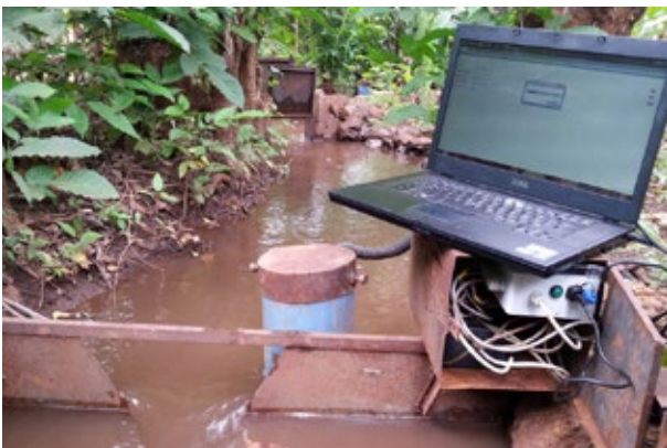
Fig. 6. Measurement of canal flow dynamics by using pressure infrared sensor installed with V-notch 60° weir.
