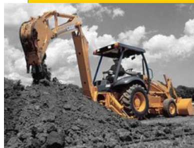
Unloading dredged material at a new location.
