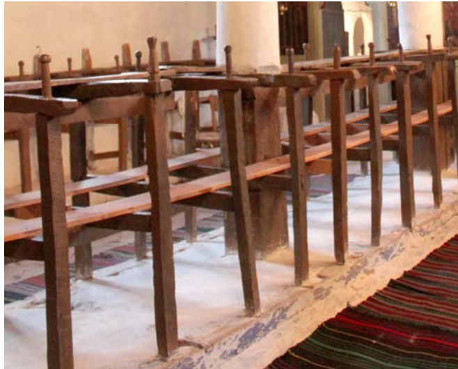
Figure 2. Old stasidia since 1820 still in use, where the original and hardly damaged moveable seats have been replaced by a stable plank (St.Taxiarches Achladoxori, Serres)
