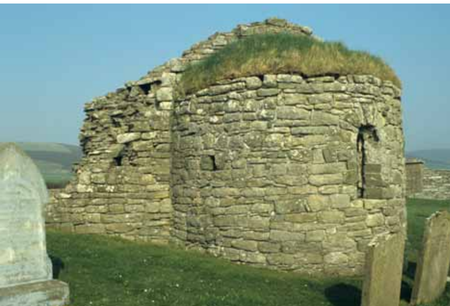
50. The Round Church, Orphir, part of a lordly estate complex © Crown Copyright reproduced courtesy of Historic Scotland.
