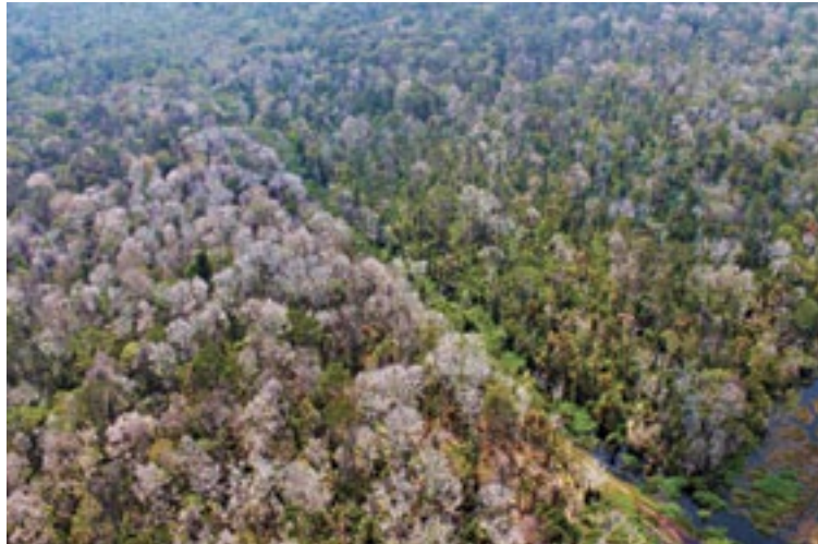
FIGURE 16 Peat swamp forest trees killed by elevated water levels caused by back-flooding of the forest as a result of the construction of adjacent bund with no culverts between the forest and agricultural land.
