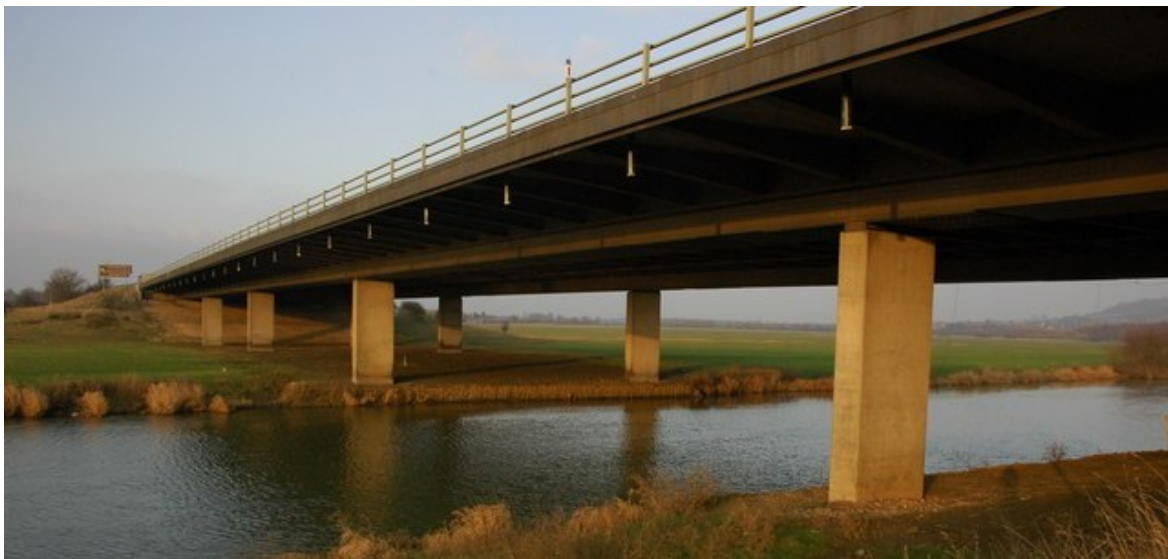
Figure 21. The M5 Motorway, which passes within 210 metres of the village, creates a serious noise nuisance for residents.
