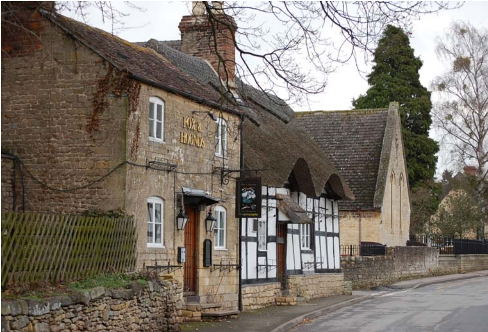
Figure 24. A group of 17 th , 18 th and 19 th century Cotswold buildings in Church Street.
