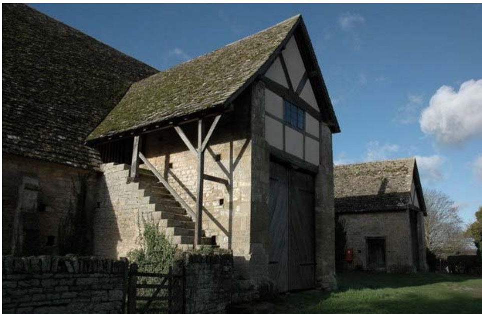
Figure 8. Bredon Barn, a 14 th century threshing barn belonging to the National Trust.
