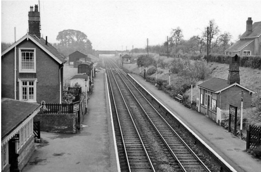
Figure 7. Bredon Station prior to its closure in 1965.
