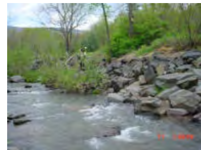
Rip Rap, looking upstream
