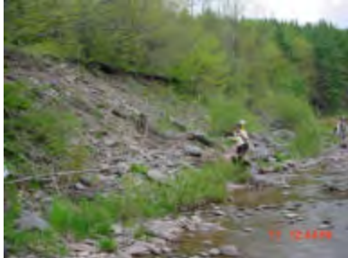
Bank erosion, looking upstream
