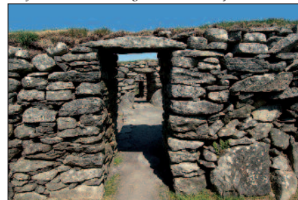
Roofless blackhouse showing lintel over doorway
