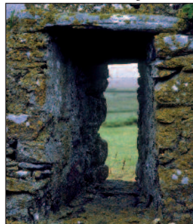
St Olav window showing narrow slit
