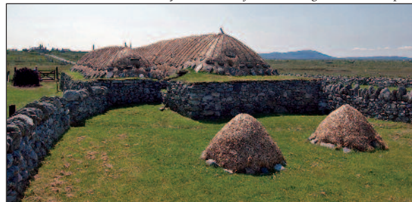
Stackyard and back of house showing barn and main part
