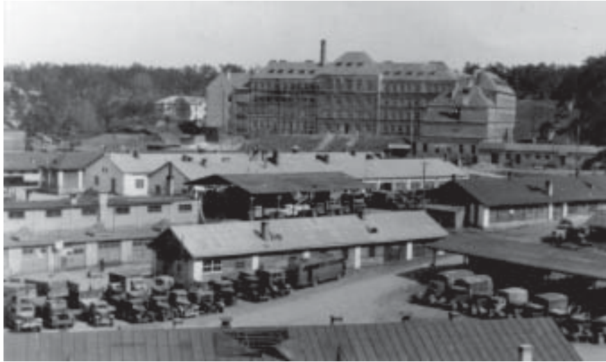
Main HKP work area in Olandu Street
