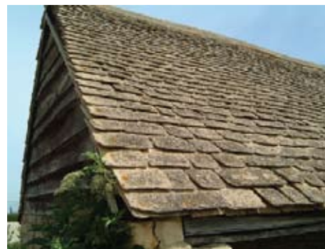
'Cotswold Slates' forming a stone roof on a Cotswold farm building
