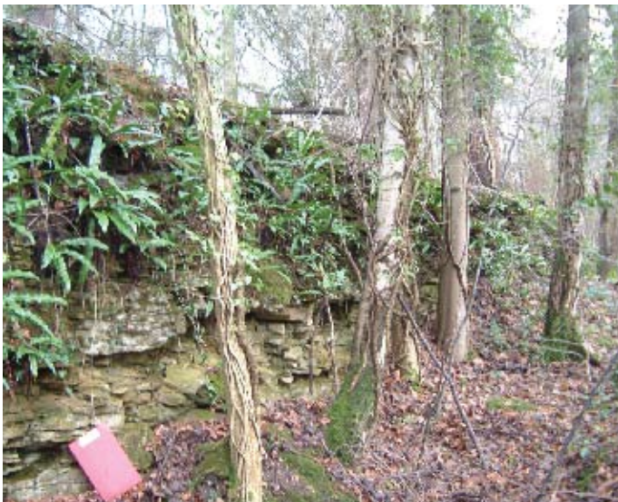
Four Mile Lodge Quarry near Cirencester. Faces are becoming overgrown and exposure lost
