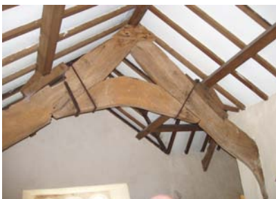
Cruck roof timbers
