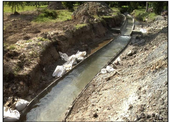
Fig. 6. The stream in Kács was dredged out after the flood in April 2010 and a concrete streambed has been built. The picture was taken on 21 August 2010.
