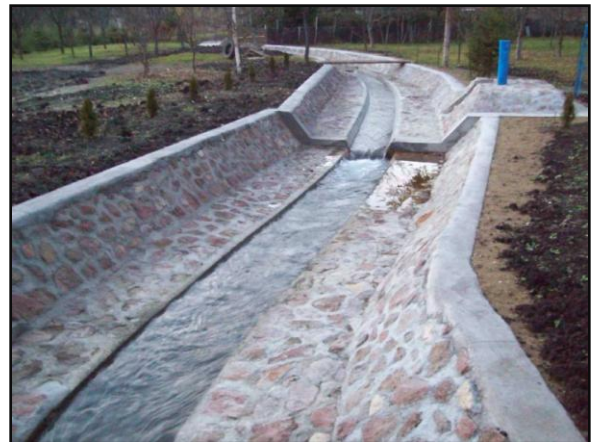
Fig. 7. The newly built concrete streambed of the stream in Kács. The picture was taken on 14 November 2010.
